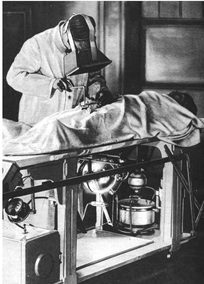
Figure 2.4: World War I surgeon uses a fluoroscope to locate bullets. X-rays from the source under the table excite fluorescent salts in the screen worn on the surgeon's face. Credit to Dr. Hoguet, American Ambulance Hospital, Neuilly, France [92] .
