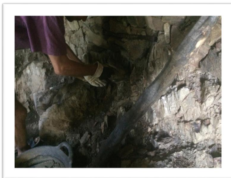
Figure 5.9: Working with cement in Can Decreix. Source: Author
