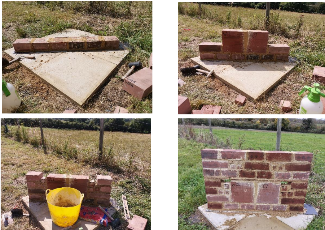
Figure 5.2 Images of wall under construction in July 2019, facing East ©Author
