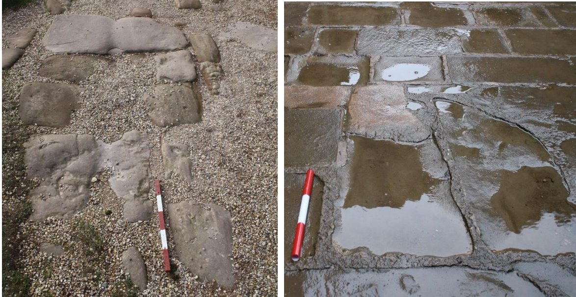
Figure 2.13 Left: Historic floor stone Type 1 with Type 4 infill, adjacent to the Norman Keep. Linear wear appears to be wheeled traffic derived. Actual age of stone is unknown. Scale 0.5m. Right: Type 2 stone. Dishing out of stone centres (note pooled water) exacerbated by inappropriate resetting of stone in high strength modern mortar. Scale 0.3m. Images © Author
