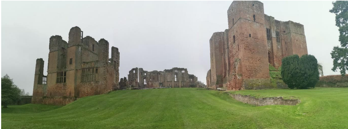
Figure 2.2 Leicester's building (left), the great Hall (centre) and the Norman Keep (Right) taken from the base courtyard. Image © Author
