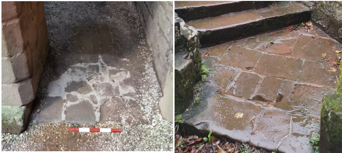
Figure 6.4 Representative Exposed Stone Flooring At Kenilworth Castle. Image ©Author
