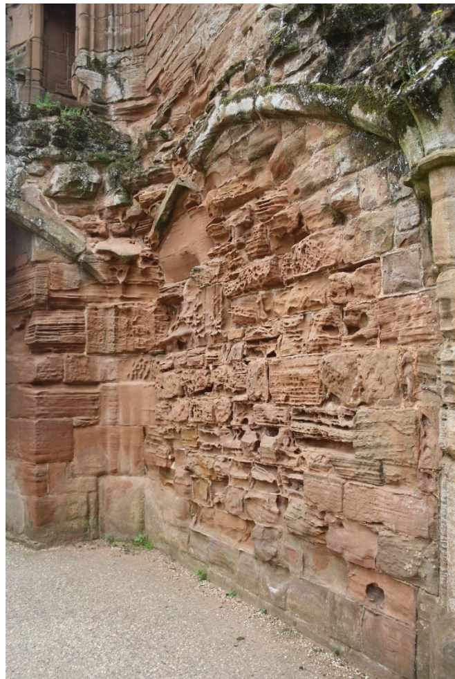
Figure 2.6 Inner wall of Great Hall showing Alveolisation caused by wind driven rain Image © Author
