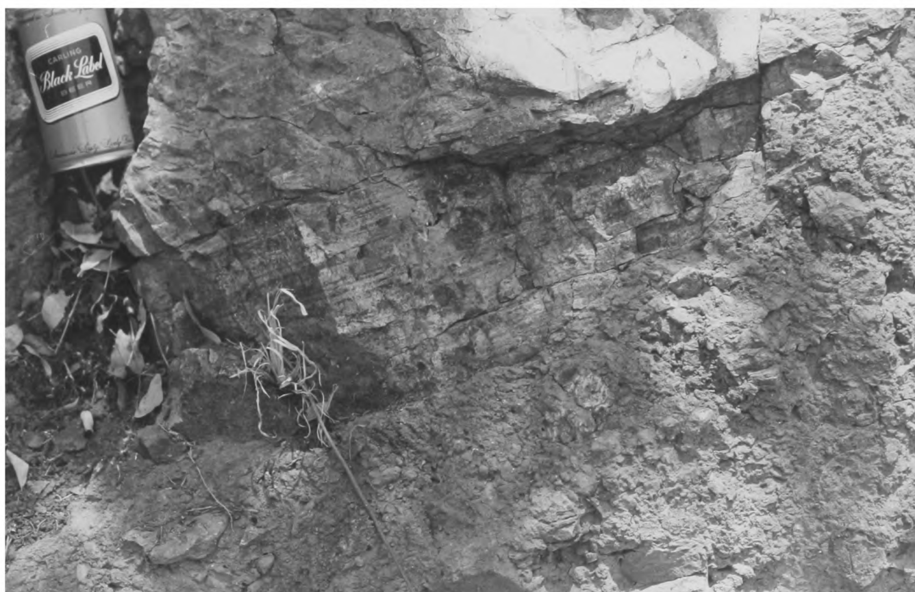
PLATE IV.31 Flow contact in road cutting 100 m west of Mozambique border, east of Komatipoort. Irregular contact of slightly banded rhyolite with pyroclastic rubble. The banding does not respond to the irregularities in the contact surface and is probably secondary, related to the joints.
