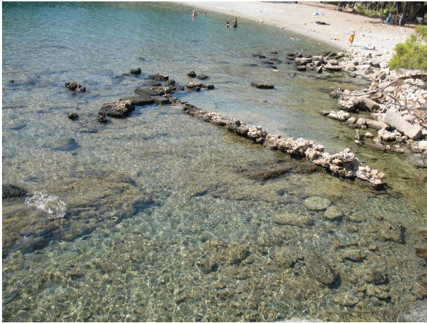
Figure 67. Sea walls in the Stadthafen (author's photo).
