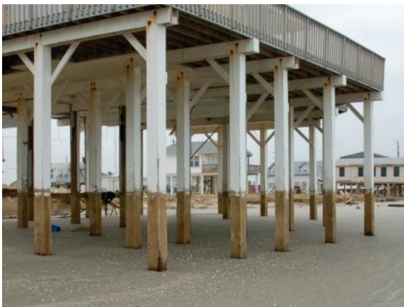
(a) (b) Figure 1.3. (a) Global scour beneath an elevated coastal building (photo credit: FEMA); (b) Local scour at a bridge pier (photo credit: USGS).
