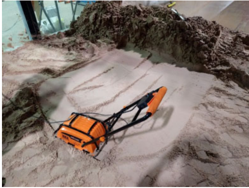
Figure 6. Compaction of sand layers using plate compactor.
