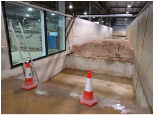
Figure 4. Pit section of the Fast Flow Facility prior to installation of the experiments.
