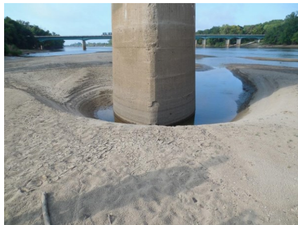
(a) (b) Figure 1.3. (a) Global scour beneath an elevated coastal building (photo credit: FEMA); (b) Local scour at a bridge pier (photo credit: USGS).
