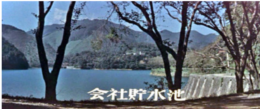
Fig. 32: The Kawachi Water reservoir in southern Yahata , where the Steelworks generated their water supply for production
