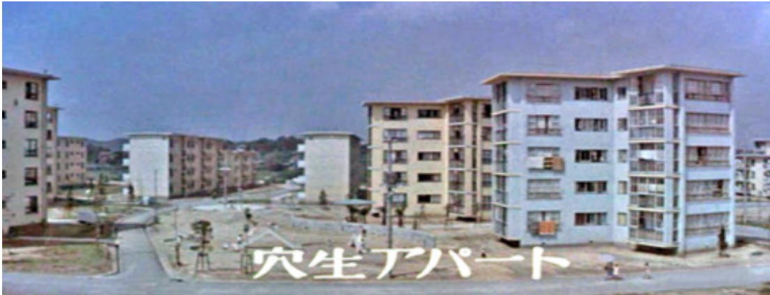
Fig. 30: Five-storied concrete buildings (Anō company housing), constructed with steel from the Steelworks
