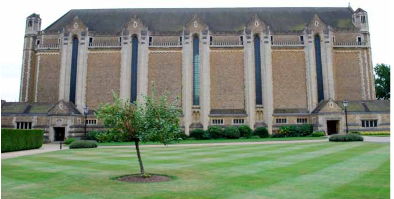
Fig. 3.61 North facade, Charterhouse Chapel (1927). Author, 2012.
