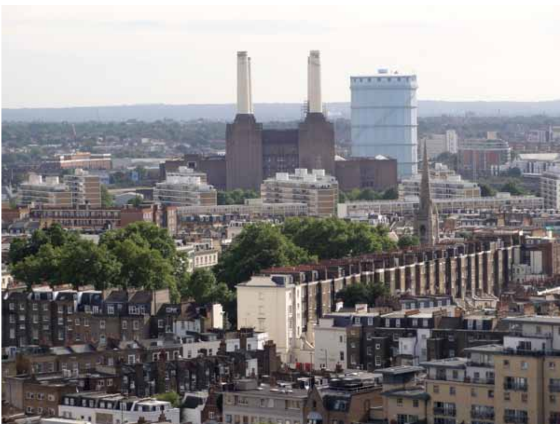
Fig. 4.16 Battersea Power Station (1932). Author, 2012.
