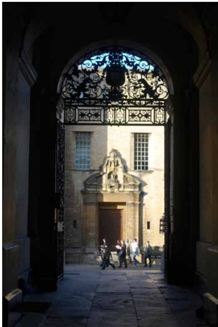
Fig. 2.20 Ceremonial Broad Street Door, New Bodleian Library, viewed from the processional axis that runs through the Bodleian Old Schools and the Clarendon Building. Author, 2010.
