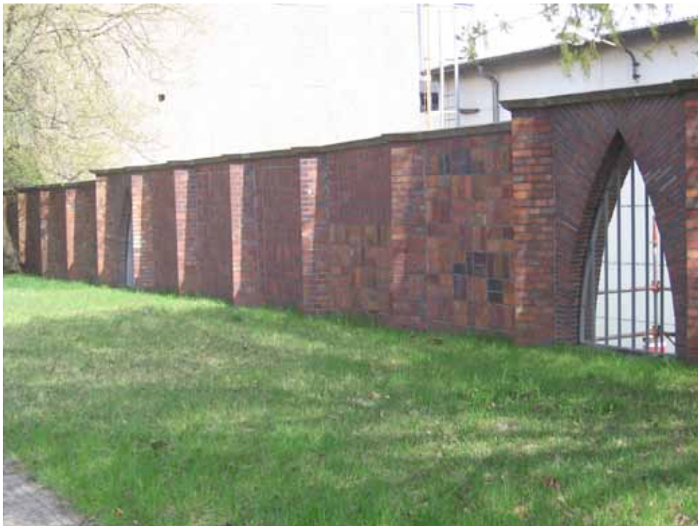
Fig. 4.41 Wall at Klingenberg Power Station, Berlin (1926), by Werner Issel. Eszter Polonyi.
