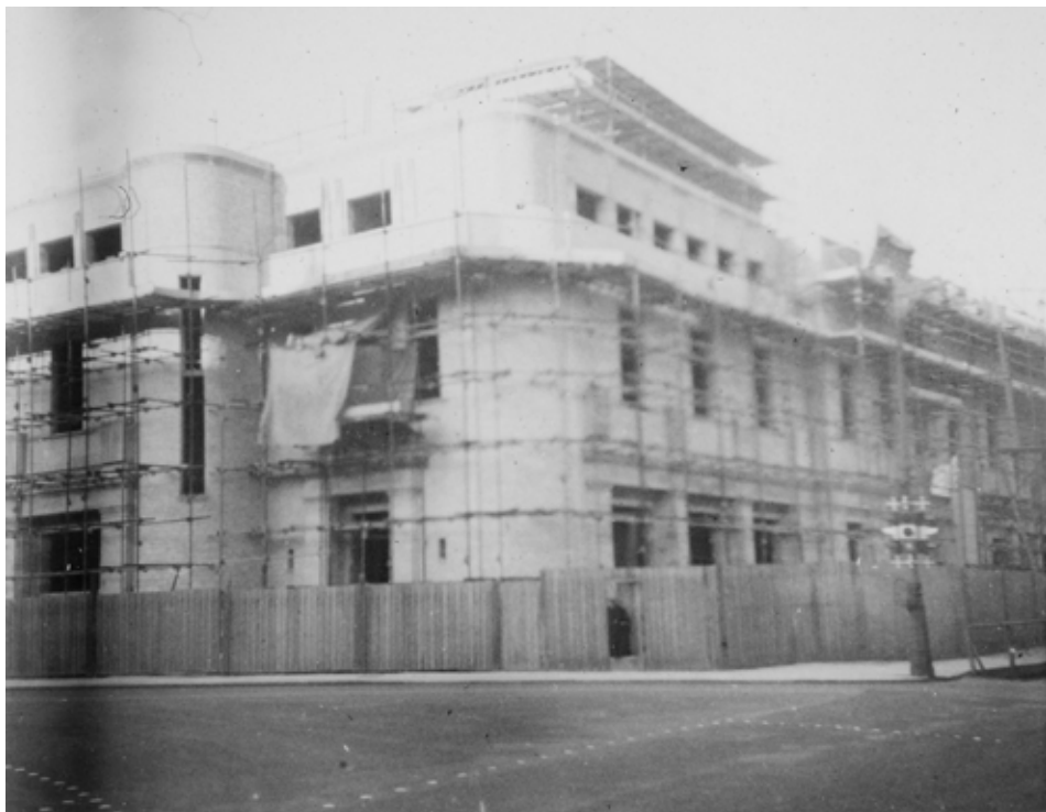
Fig. 2.29 The New Bodleian under construction, c. 1937. Bodleian Library.
