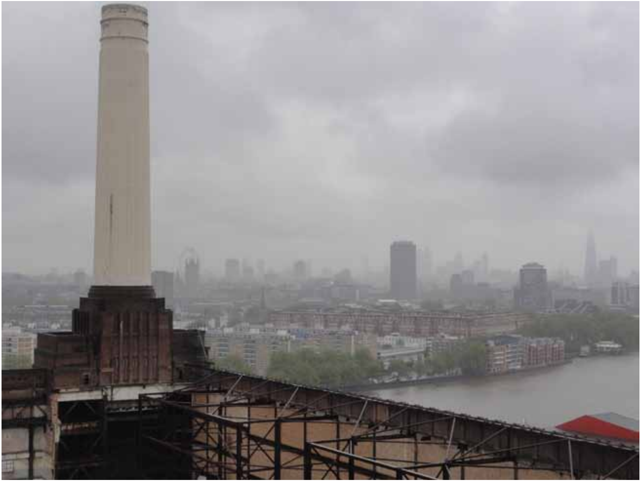
Fig. 4.42 A chimney of Battersea Power Station. Author, 2012.
