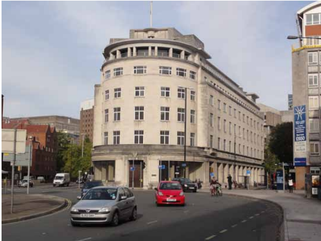
Fig. 4.2 Bristol Electric Company Headquarters, Bristol (1939). Author, 2011.
