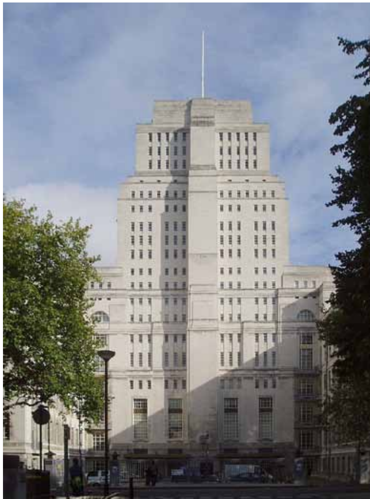
Fig. 2.5 University of London Senate House, which includes the library (1937), by Charles Holden. Steve Cadman.
