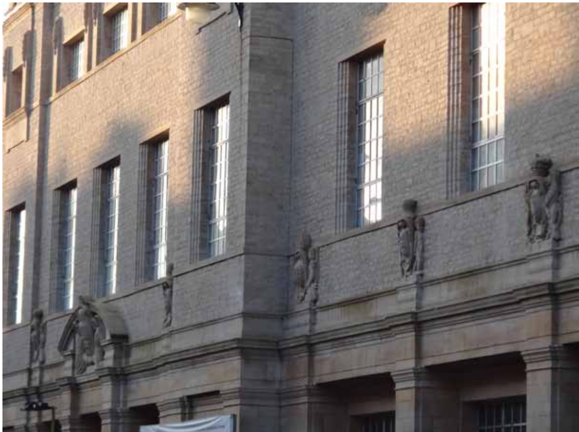
Fig. 2.35 Detail of the Parks Road façade of the New Bodleian, showing the placement of carved ornament. Author, 2013.
