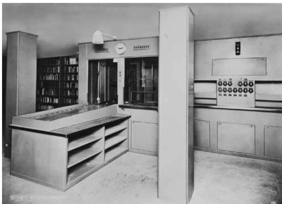
Fig. 2.21 Conveyor Belt Station, New Bodleian; photograph dated 1942. Bodleian Library.
