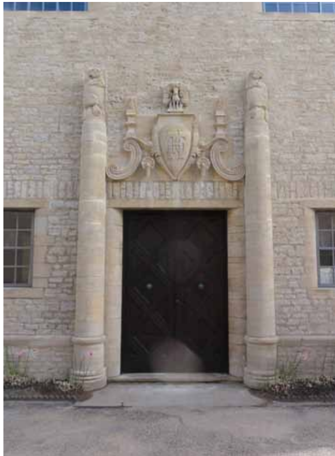
Fig. 2.32 West entrance to Hartland House. Author, 2012.
