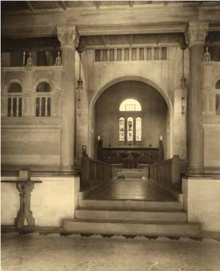
Fig. 1.34 Interior of Whitelands College Chapel. RIBA.
