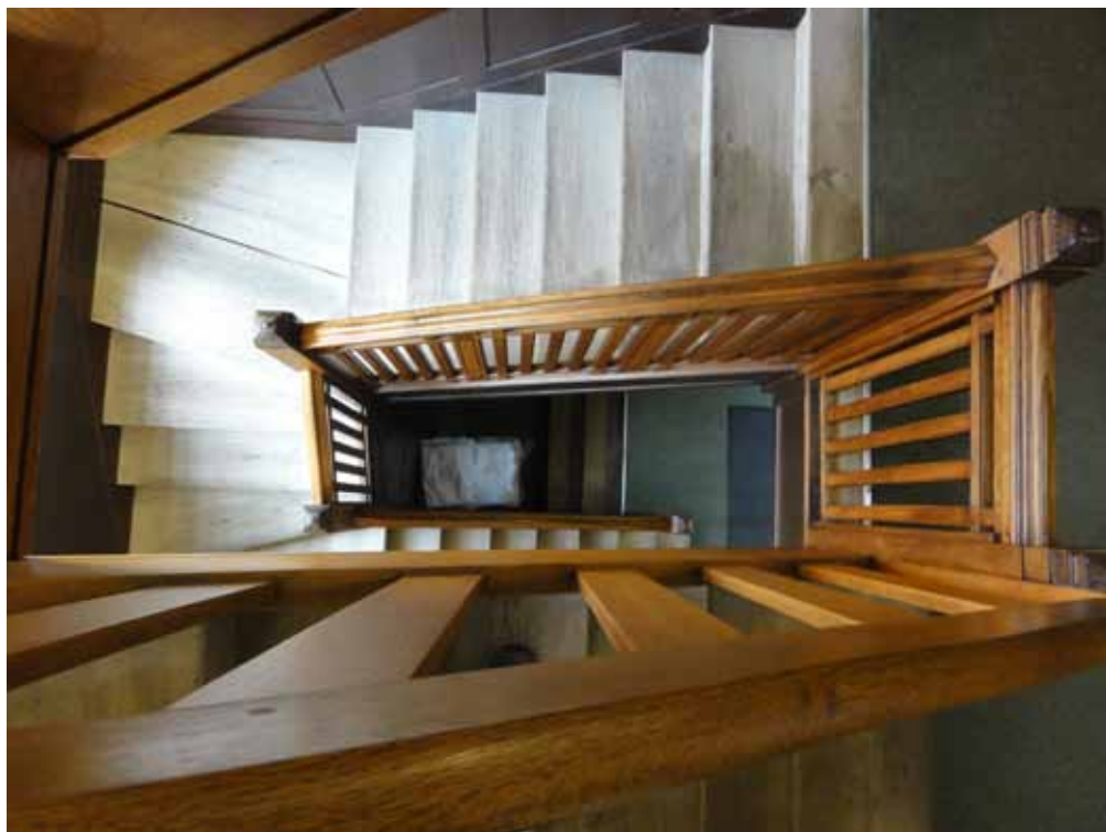
Fig. 1.4 Internal staircase, Memorial Court, Clare College, Cambridge. Author, 2011.
