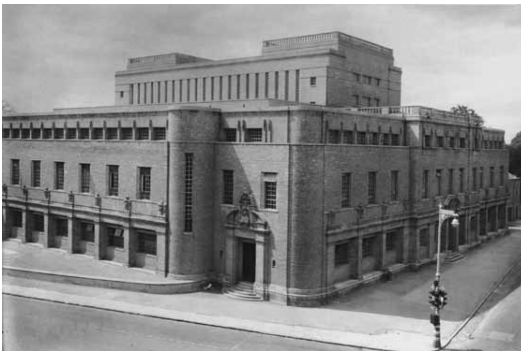
Fig. 2.17 New Bodleian Library, photographed shortly after completion. Bodleian Library.
