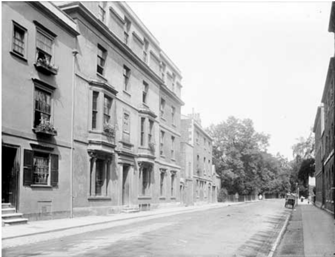
Fig. 2.28 View of Parks Road before the construction of the New Bodleian, with Ripon House at centre, near the location of what would become the library's main entrance. Bodleian Library.
