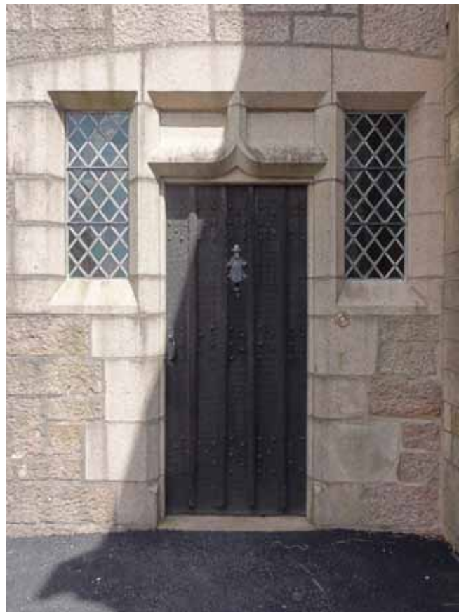
Fig. c.4 Detail of adzed door, St Columba's Cathedral, Oban (1934). Author, 2011.
