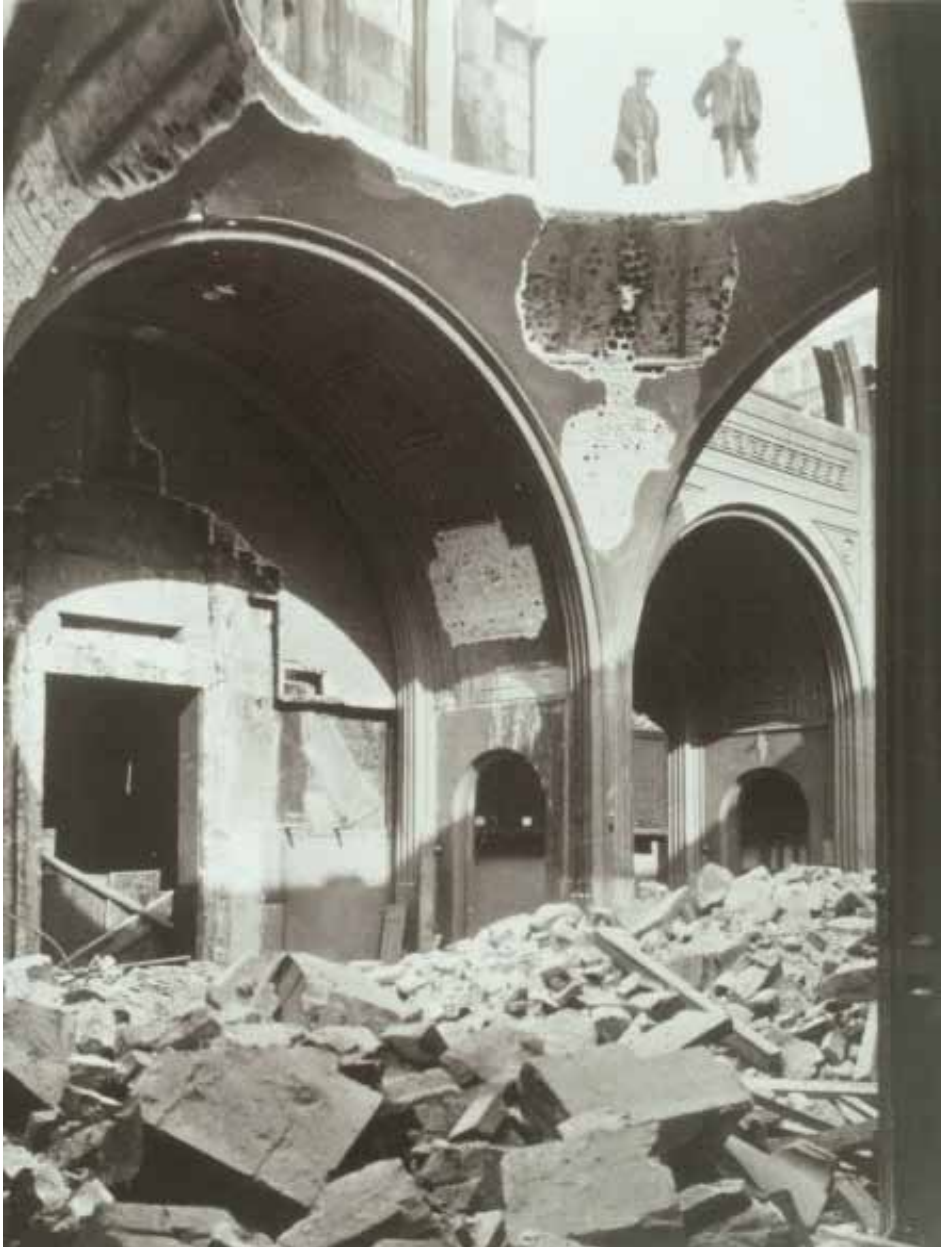
Fig. 1.11 Demolition of John Soane's Bank of England c. 1926. F R Yerbury, The Old Bank of England , (London, 1926).
