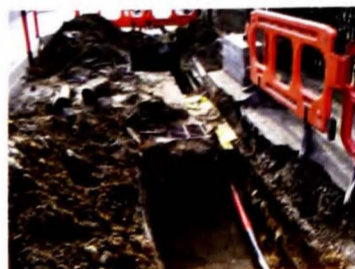
P: Gas reconnected N: Gas reconnected
