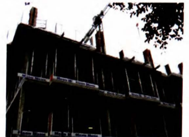
P: Fulfilling work N: Disruption
