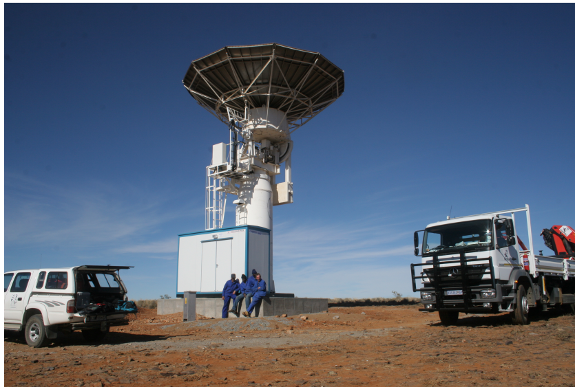
Figure 3.25: The final destination for C-BASS South at Klerefontein together with a number of the HartRAO team involved in establishing the site and installing the antenna.
