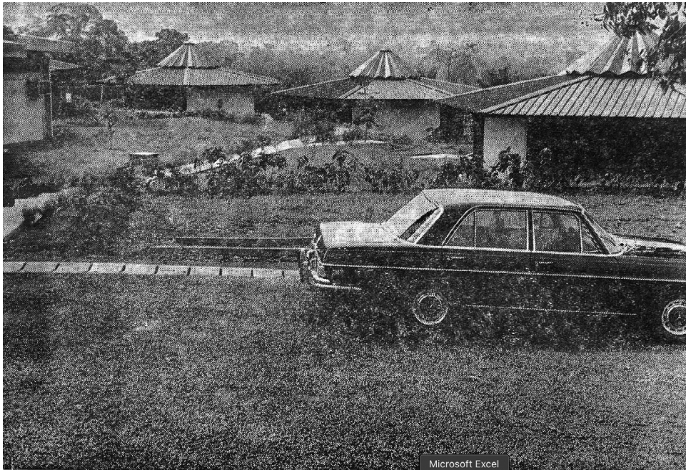
Figure 1: IRIC buildings on the campus of the University of Yaoundé 6 (source: IRIC Brochure, Graduate Institute Archive, Geneva, HEI 2431; reproduced by permission of the International Relations Institute of Cameroon)
