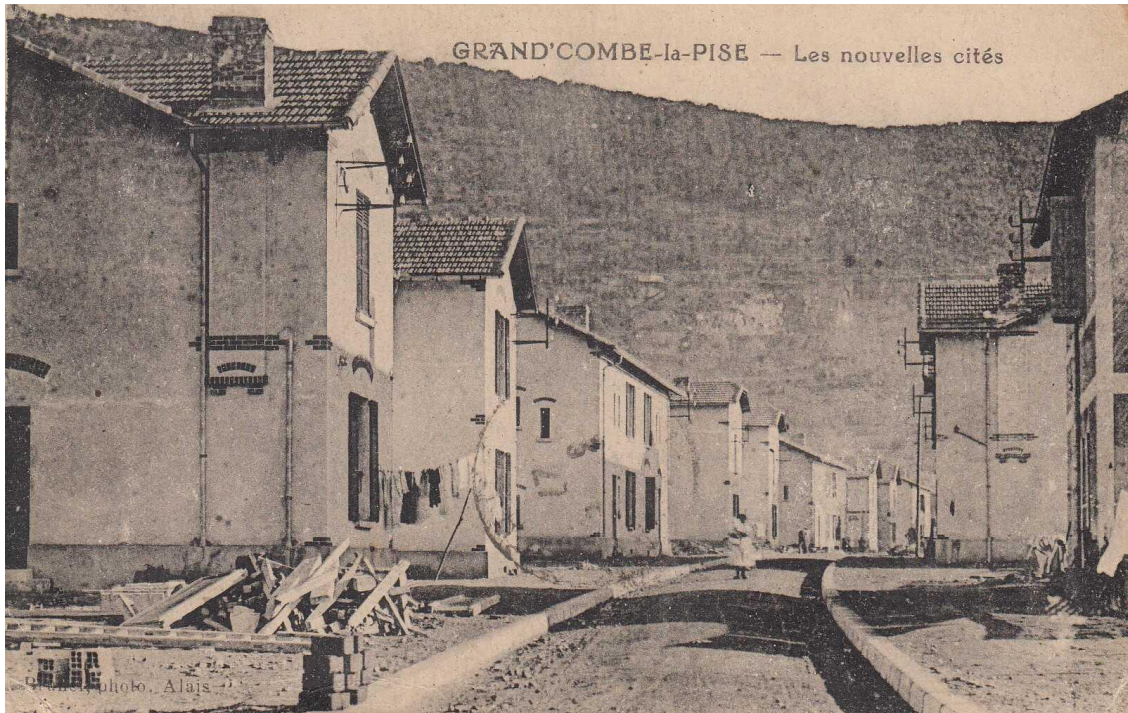
Figure 3-1 AMA 5FiGC12, New housing development in La Grand'Combe, 1923
