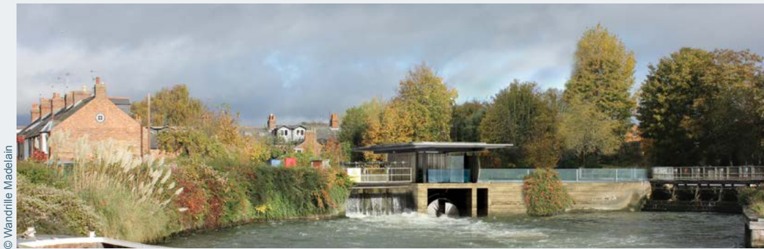
Figure 8.3 Osney Lock Hydro: an example of community crowd-funding in Oxfordshire
