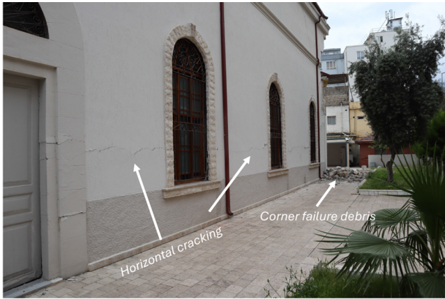
(a) South façade.
