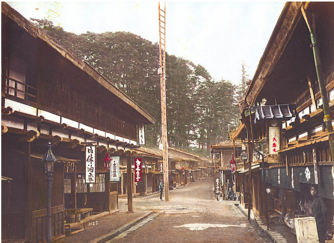
Figure 12: 'Shimono Suwa (Tea House) and Fire Bell at Nakasendo', from a collection of images of the Nakasendō taken by the documentary photographer Kusakabe Kimbei (1841-1934) during the early Meiji period.
