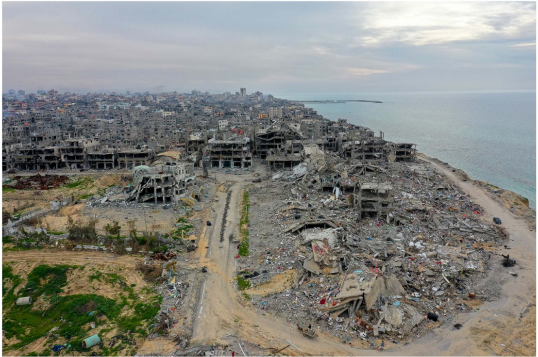
Figure 1. View of destruction in northern Gaza, February 2024. Credit: Abdullah Al-Haj / UNRWA, used with permission.
