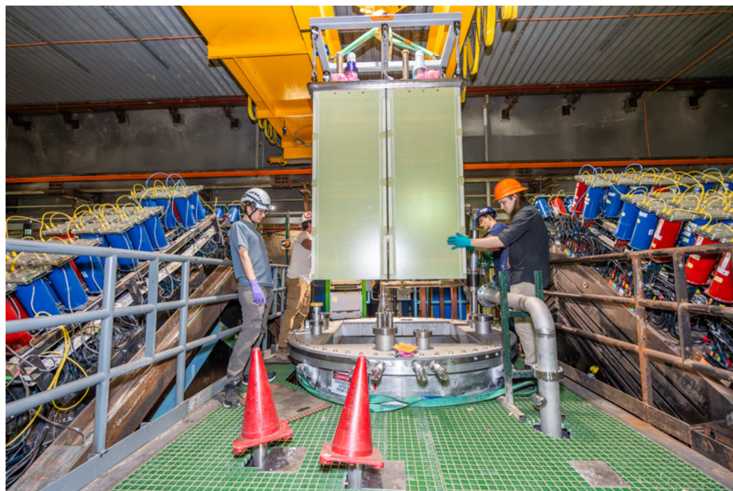
Figure 8. Installation of the 2x2 module array in the MINOS Underground Hall on 23 October 2023 [43].
