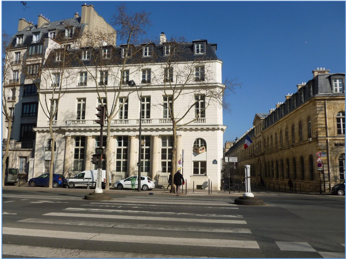
Figure 1.2 - Maison Brongniart , Blvd des Invalides, Paris. Constructed 1781. Alexandre-Théodore Brongniart. Photo: J. Carr-Trebelhorn, 2016
