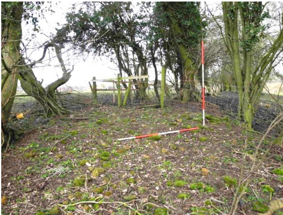
Figure 71. Hanwell, collapsed remains of wall on north side of garden looking north.
