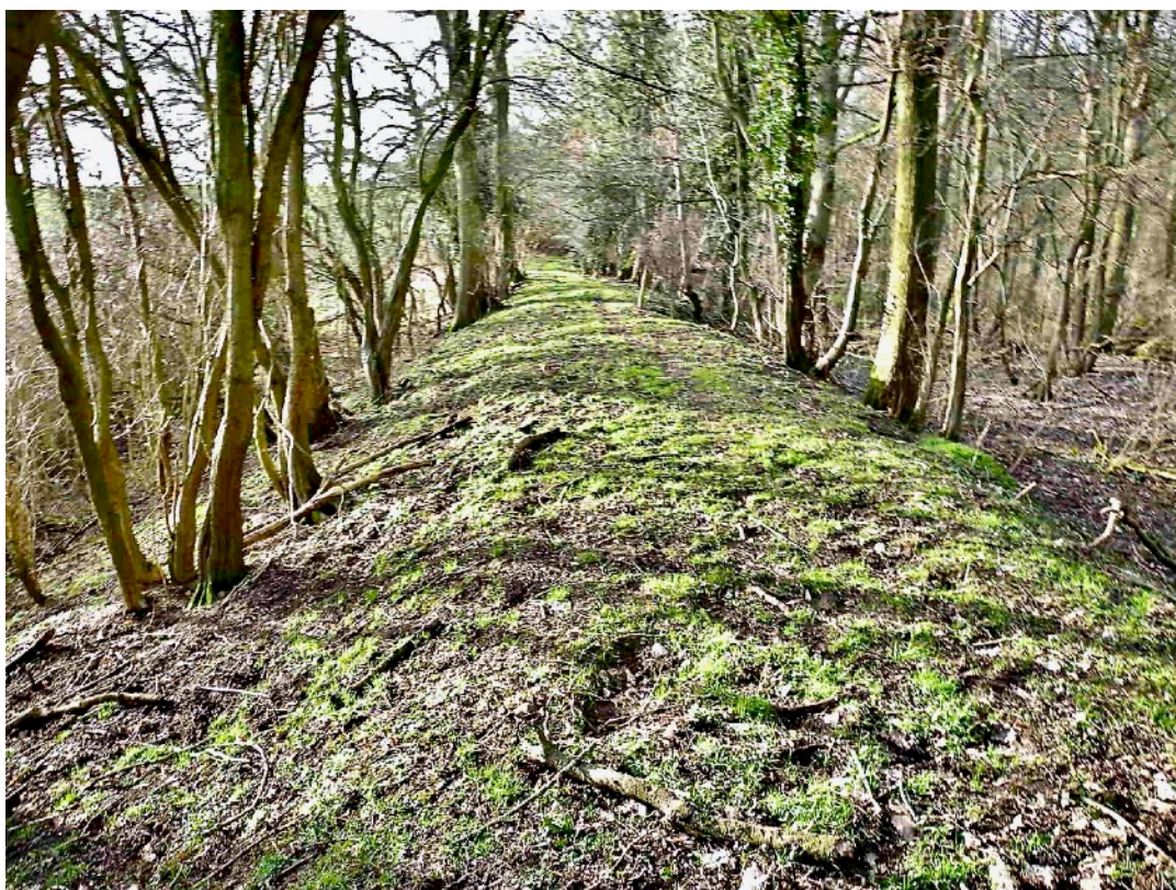
Figure 70. Hanwell, dam (Pond F) at south east end of park looking west.
