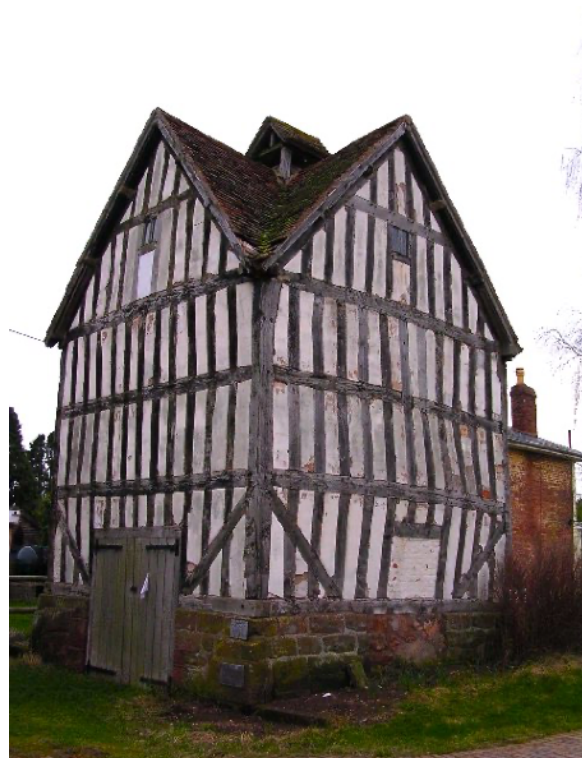
Figure 123. Hawford, Worcestershire, square timber frame dovecote.
