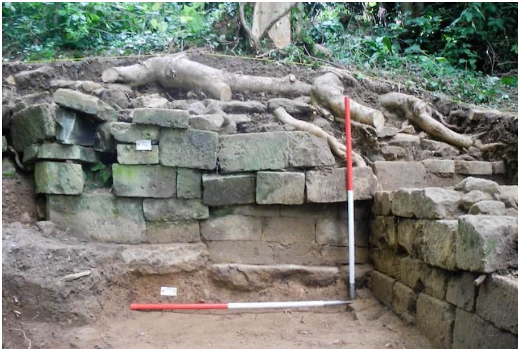
Figure 65. Hanwell, HANG14, terrace walling and base of stair looking west.
