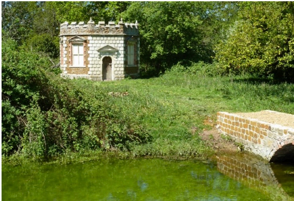
Figure 36. Hunstanton Hall, The Octagon: bridge, moat and banqueting house.
