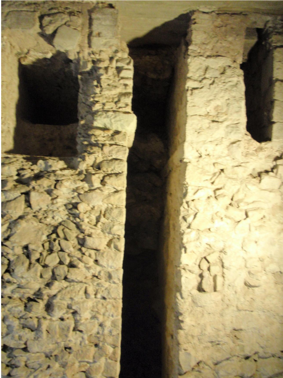
Fig. 3.6 – Barcelona: The two conduits (Colserolla to the left and Moncada to the right) inside the Casa del Arcediano.
