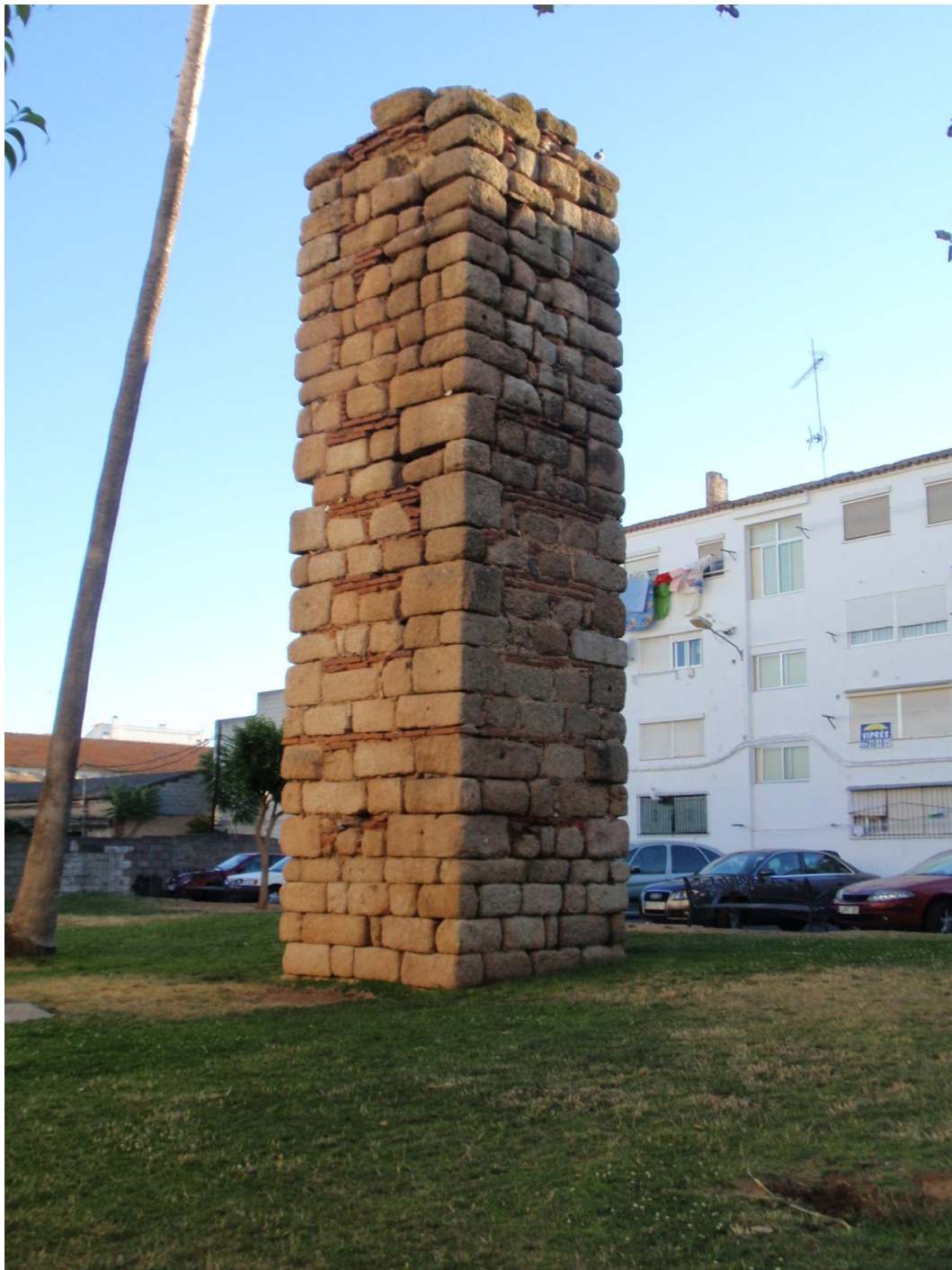
Fig. 3.39 – Mérida: Late antique (Visigothic?) pillar of the Proserpina/Los Milagros aqueduct, built with the remains of previously collapsed pillars, trying to imitate the granite and brick pattern of the other arches. Note how it is not properly straight and slightly twisted.
