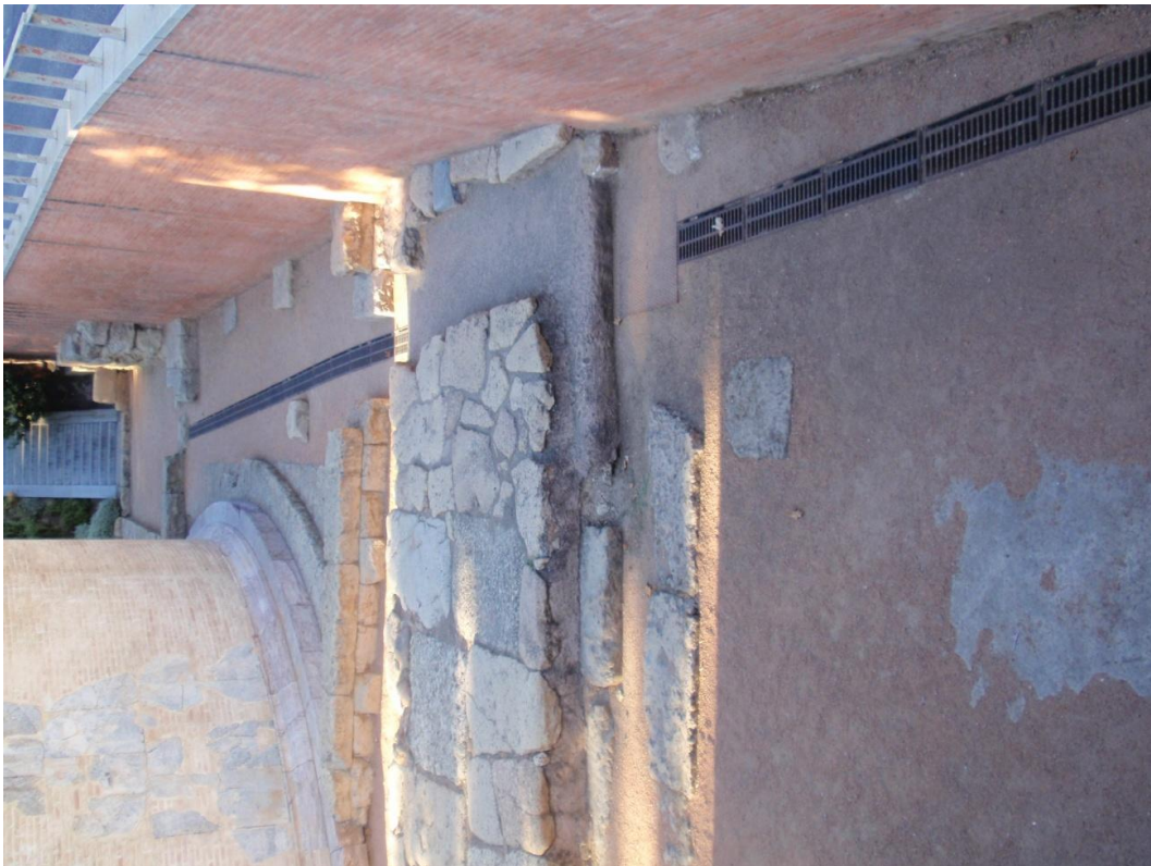
Fig. 3.26b – Córdoba: Remains at the Puerta de Gallegos in 2012: the Alcázar conduit has been preserved and is now covered by a metal grid.
