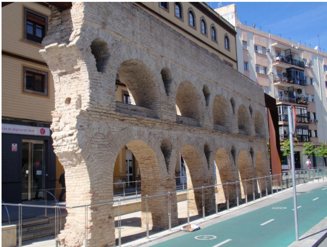
Fig. 3.87 – Seville: Standing remains of the aqueduct, probably Almohad in date (12 th -13 th c.).
