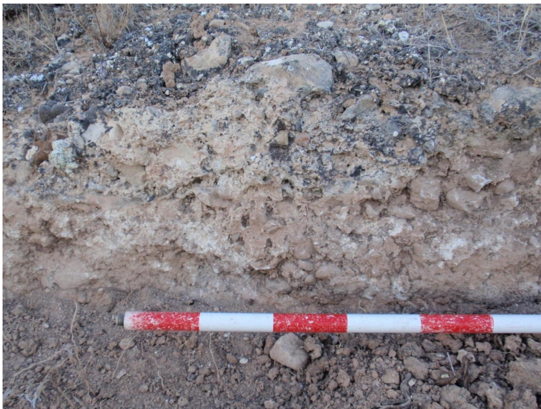
Fig. 3.71 – Reccopolis: Mortar covering the walls of the aqueduct, identified at La Paeriza 1.1.
