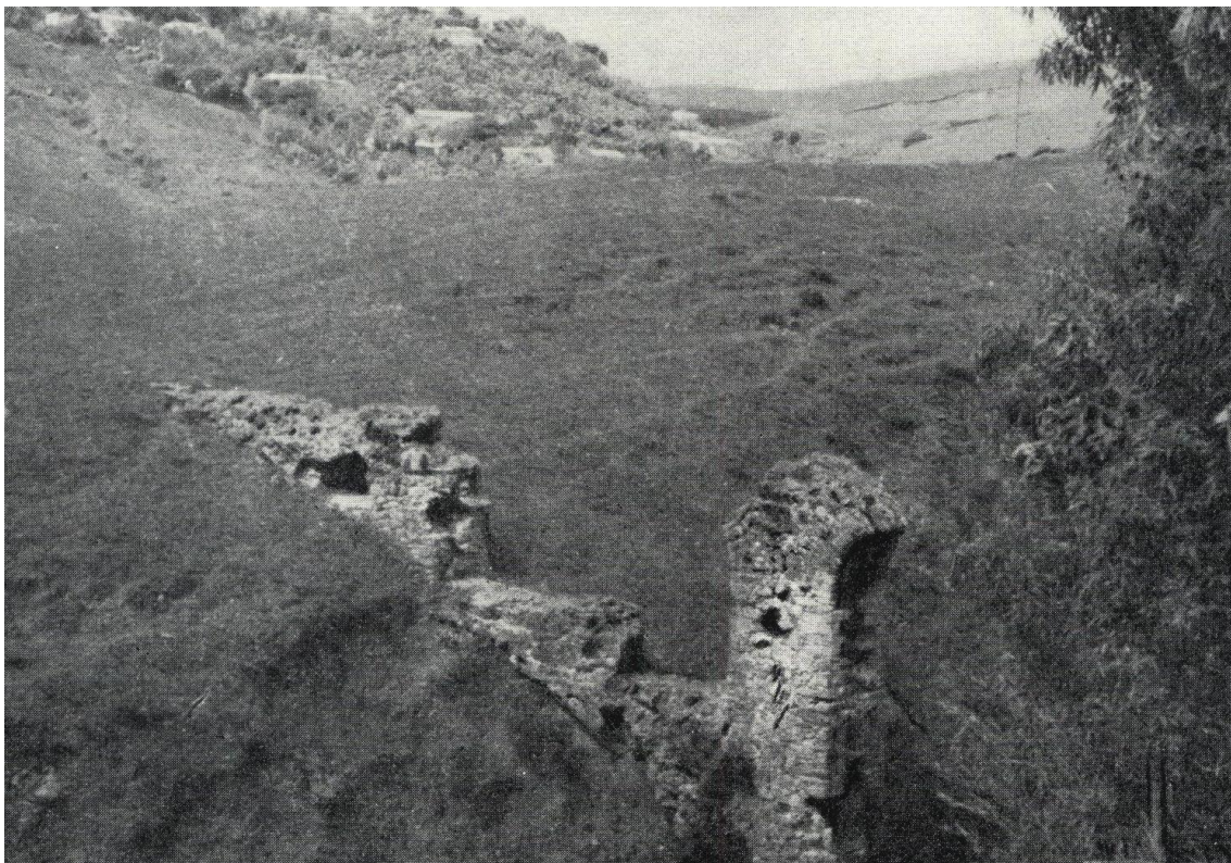
Fig. 3.103 – Ceuta: Last standing remains of the aqueduct at the Arroyo de las Colmenas (Posac Mon 1977: lám. 1).
