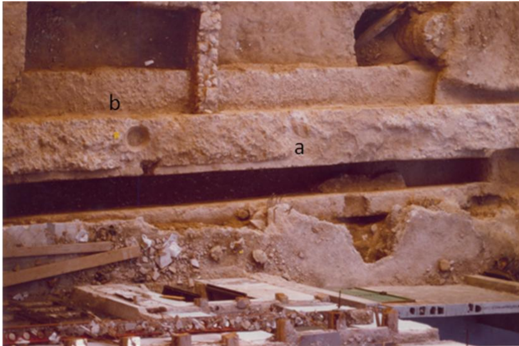
Fig. 3.78 – Valencia: View from above of section of the aqueduct excavated at Carrer Quart (Herrerros Hernández 1996: 38). The specus is clearly visible, and note the two walls built on the north side (a and b) to buttress the conduit into the slope. Wall b has been lowered in medieval times to fit new structures.
