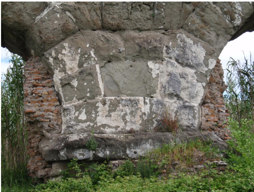
Fig. 2.4 – Sixth-century opus vittatum repairs to one of the aqueducts of Rome.
