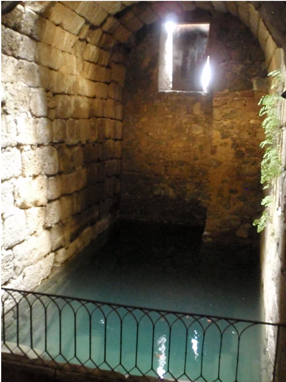
Fig. 6.9 – Mérida: Photograph of the inside of the cistern.
