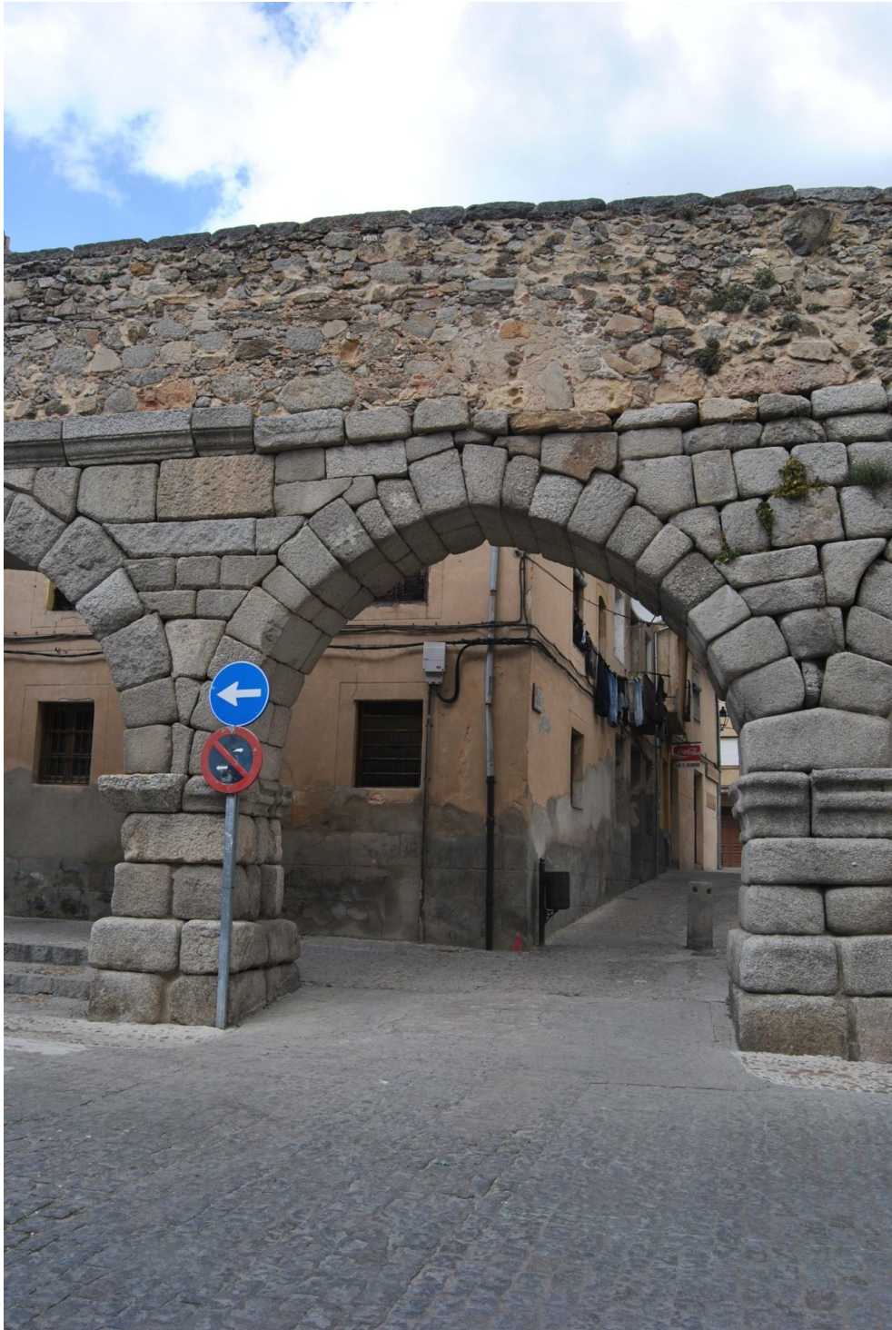
Fig. 3.58 – Segovia: Gothic arch at the aqueduct, evidence for a fifteenth-century restoration.
