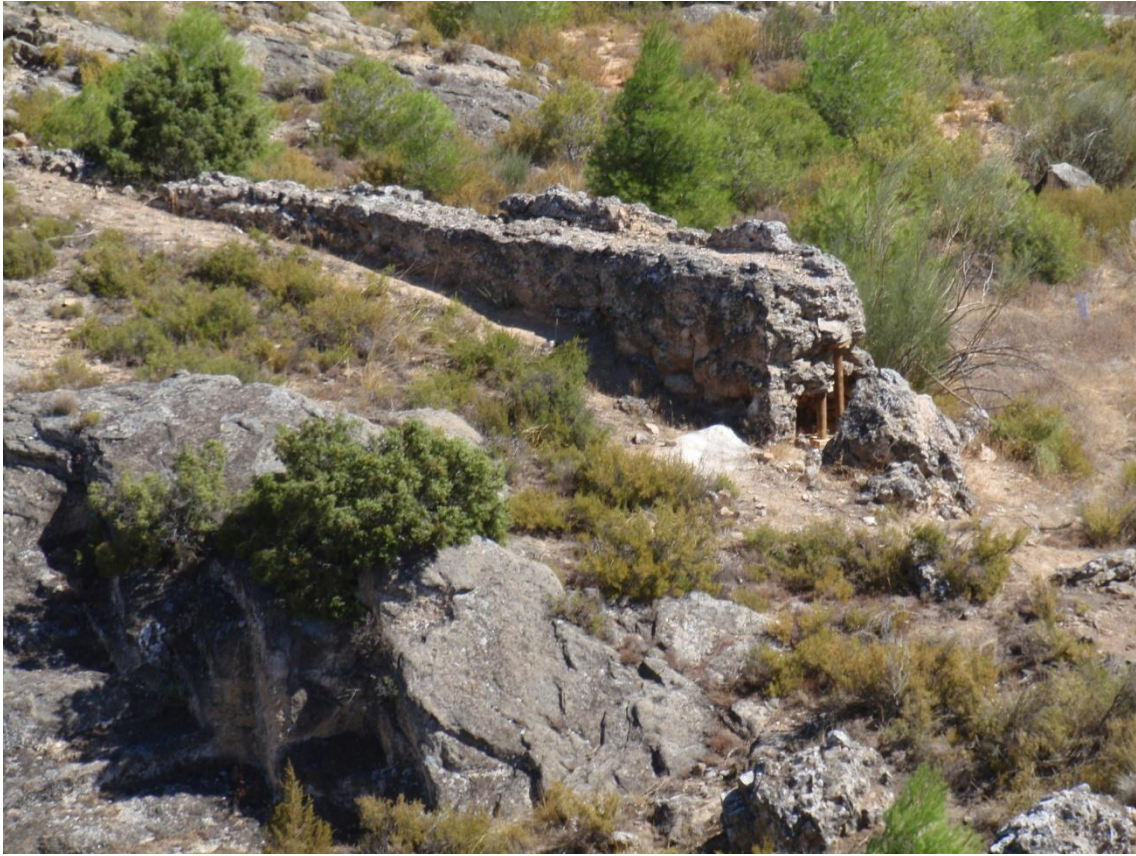
Fig. 3.66a – Reccopolis: Remains of the aqueduct at Boneta 1.1
