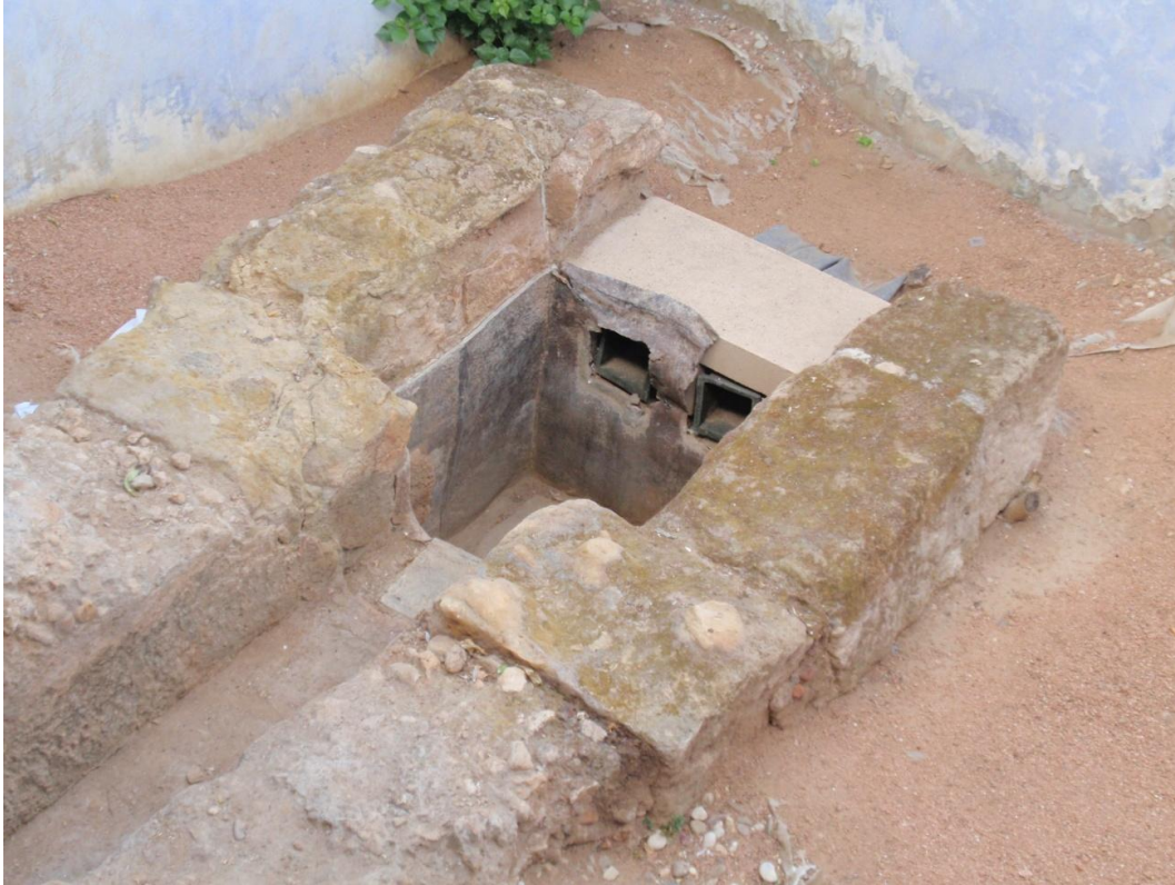
Fig. 3.20a – Córdoba: Western aqueduct distribution tank, lined with a reused lead sarcophagus and two square pipe outlets.
