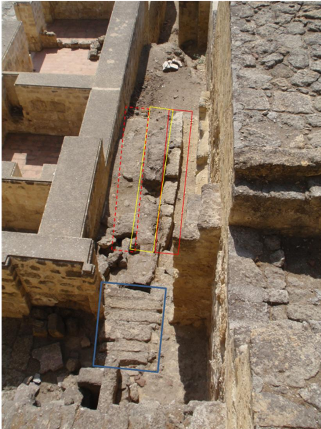
Fig. 3.18 – Córdoba: Islamic aqueduct of Madinat al-Zahra, diverted out of the old Roman aqua augusta . At the bottom of the image, the aqueduct and its covering slabs are preserved (blue), but soon both the covering slabs and even the ashlar blocks of the conduit (red) have been removed, leaving visible only the infill of the conduit (yellow).
