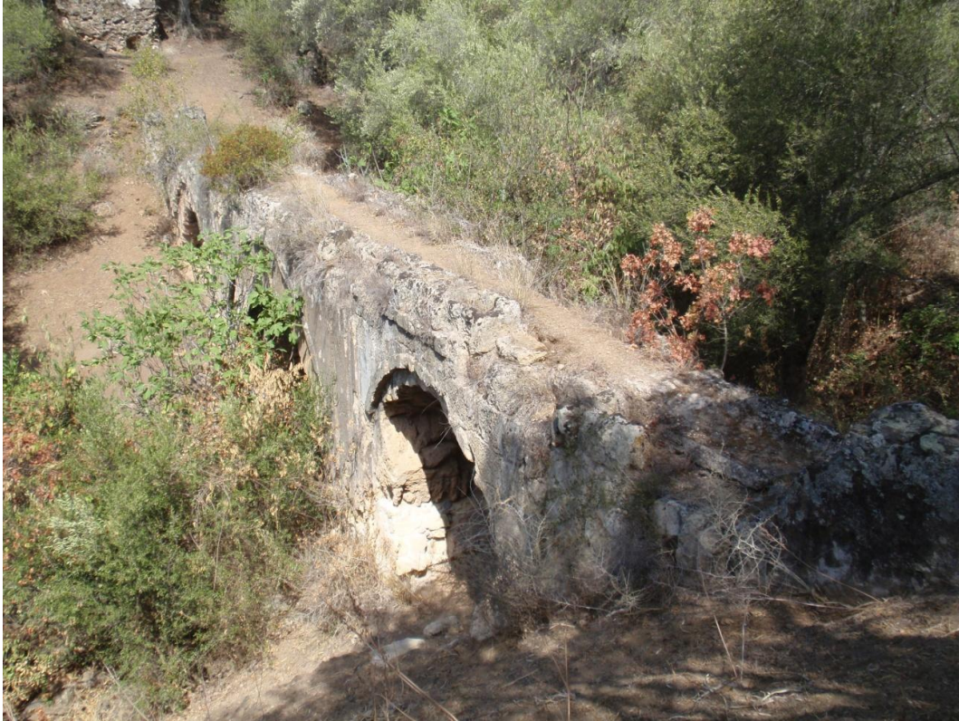
Fig. 3.28 – Córdoba: Valdepuentes Umayyad aqueduct, near Madinat al-Zahra.
