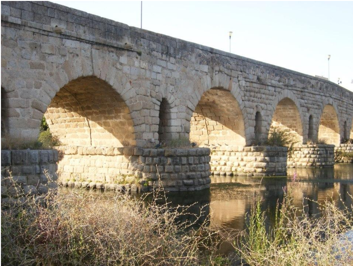
Fig. 5.2 –Mérida: the first arch on the left is considered to be part of the Visigothic reconstructions mentioned on ICERV 363:
