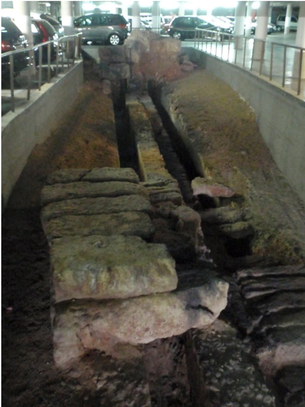
Fig. 6.4 – Córdoba: Mosque conduit built by al-Hakam II, diverted from the Western aqueduct. The conduit at a higher level is the old Roman aqueduct; the conduit at a lower level, to the right is the Islamic one. Notice how a diversion tower has been built to divert the water (see fig. 3.12)
