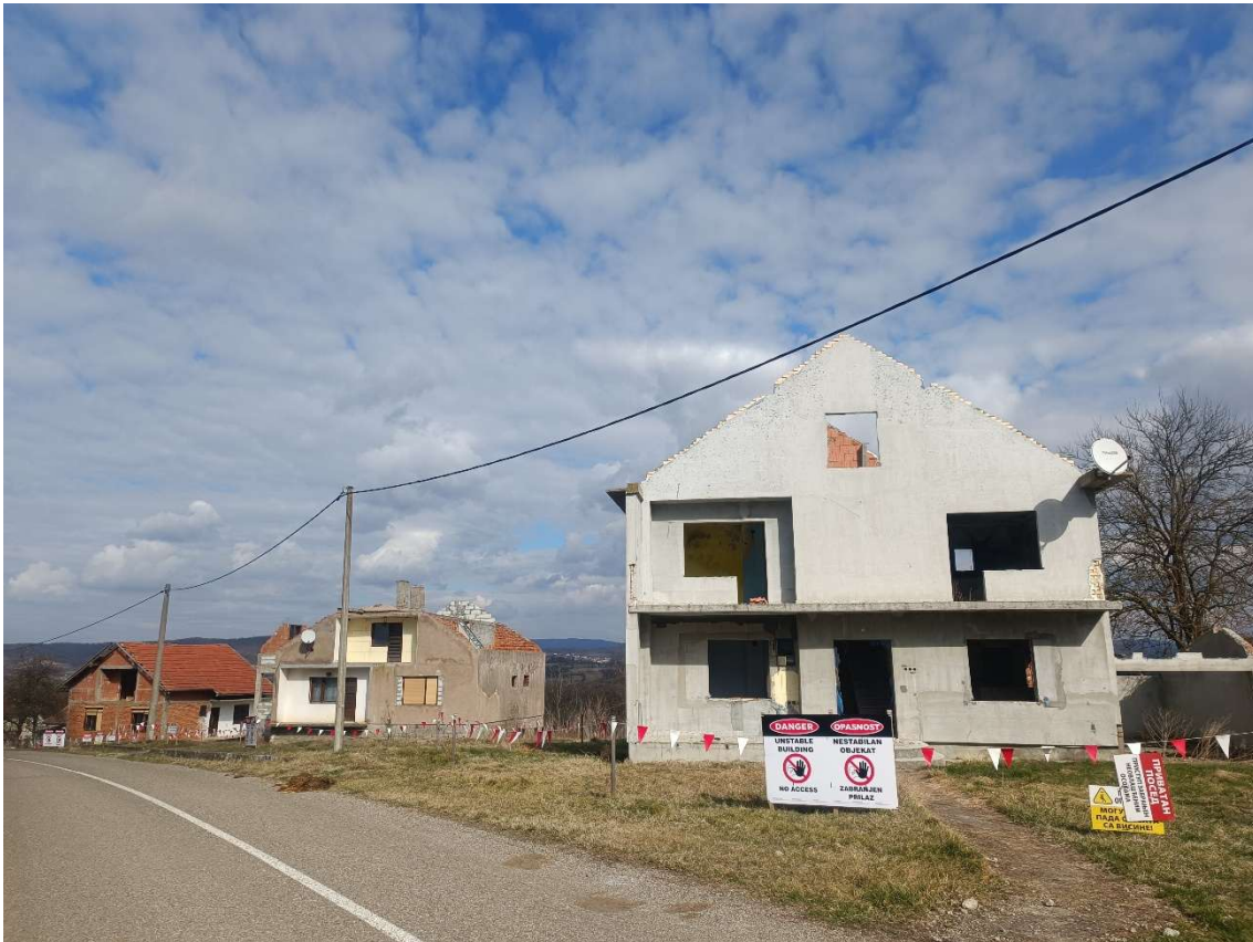
Figure 12: Houses in the Jadar Valley bought by Rio Tinto. Picture my own, February 2024.
