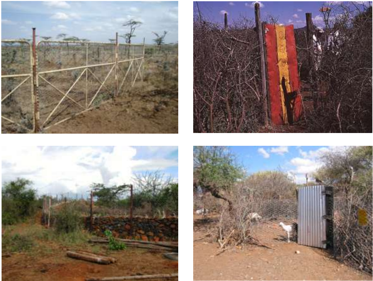
Fig 2.2. Photographs of boma wall construction in the study area a) mobile boma, b) thorn boma, c) stone boma (temporarily reinforced with chainlink until cactus planted on the top grows), and d) chainlink reinforcing weak thorn walls.
