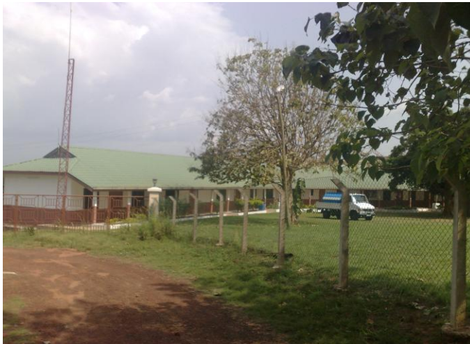
Plate 6.7.1 Administration block for local university
