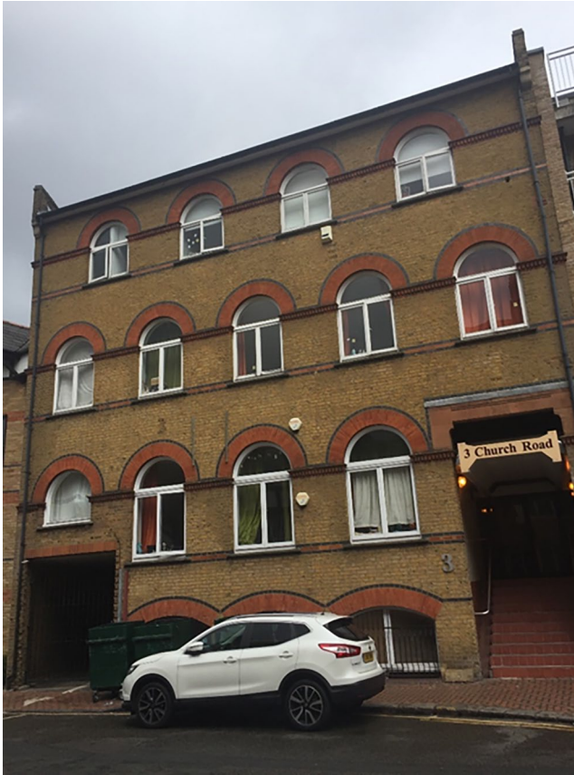
Figure 2. 3 Church Road, Croydon: an office-to-residential conversion in Croydon borough illustrating some of the uncertainties around EPC data.
