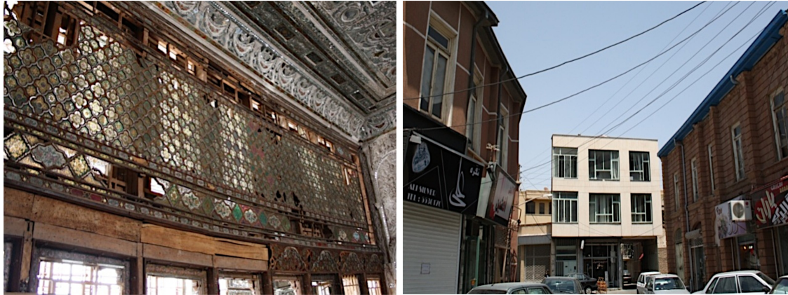
Figure 4.15: Left to right: a traditional window opening to the courtyard in Imam Jom'eh house. Tehran, Iran. Photo by the author. 2011.
