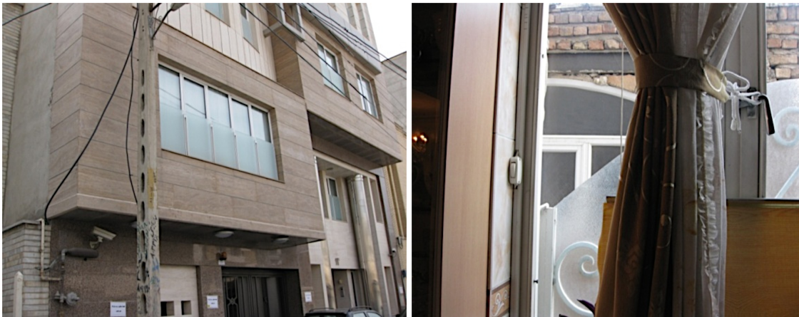
Figure 4.22: Left to right: a residential building with a half matt glass in front of the main windows. Tabriz, Iran. Photo by the author, 2013.
