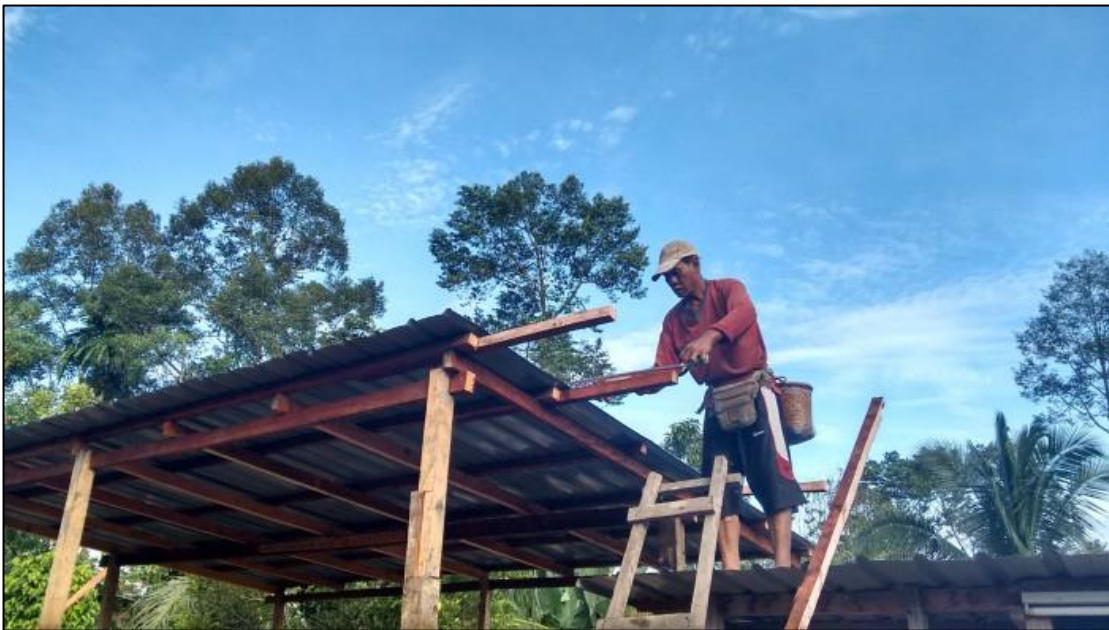
Figure 21: Apai building the solar shed (December 2015).
