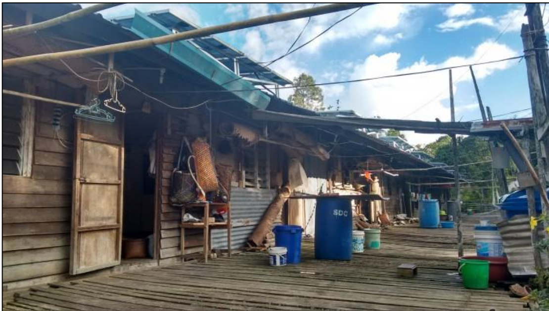
Figure 22: Merging the new (solar panels) and the old (longhouse wooden architecture, December 2015).
