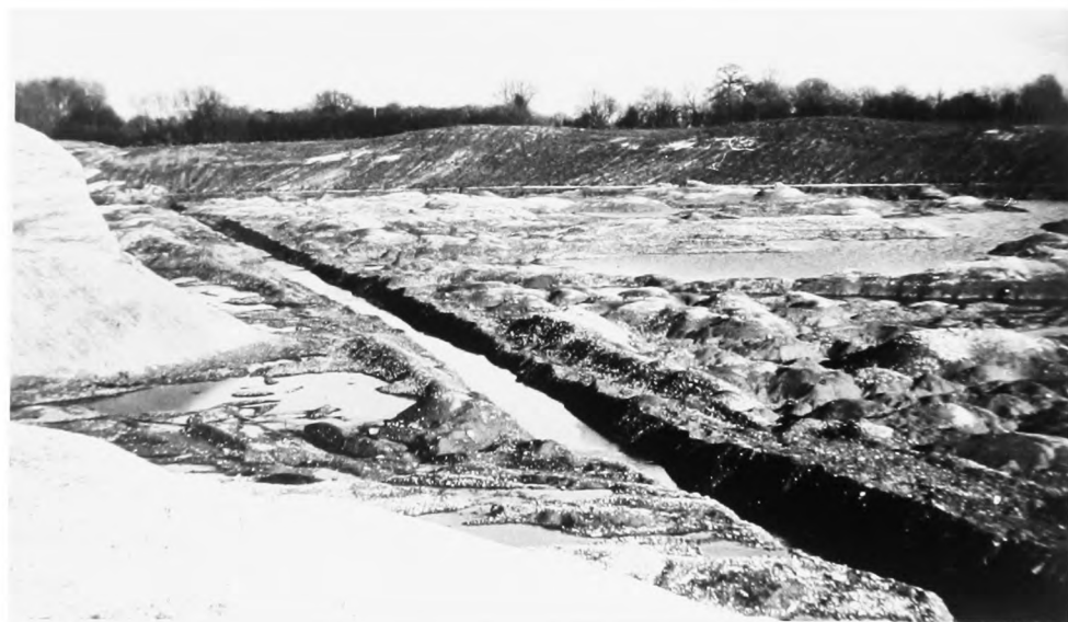
Plate 11.1 Collector ditches excavated in Oxford Clay in the bottom of Wadham-Brasenose Pit, Hardwick.
