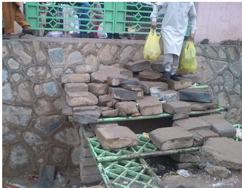
Figure 1.3 Temporary exit from Produce Market - Photograph by Laila
