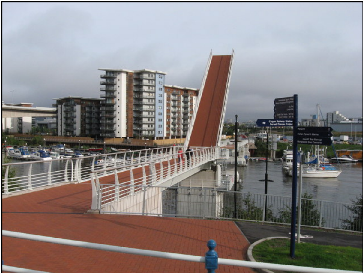
Figure 2.4: The Pont-y-Werin in the “open” position
