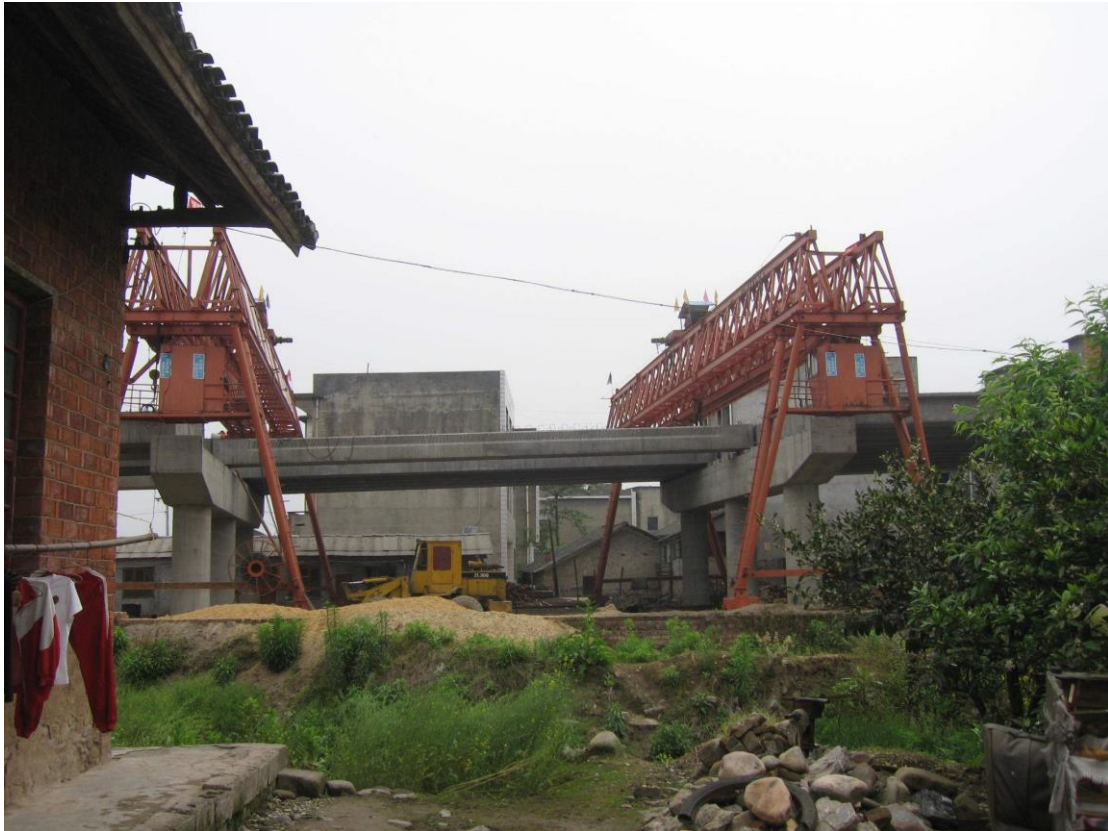
Figure 6.12 The Li River Bridge construction in Taiping village in 2009
