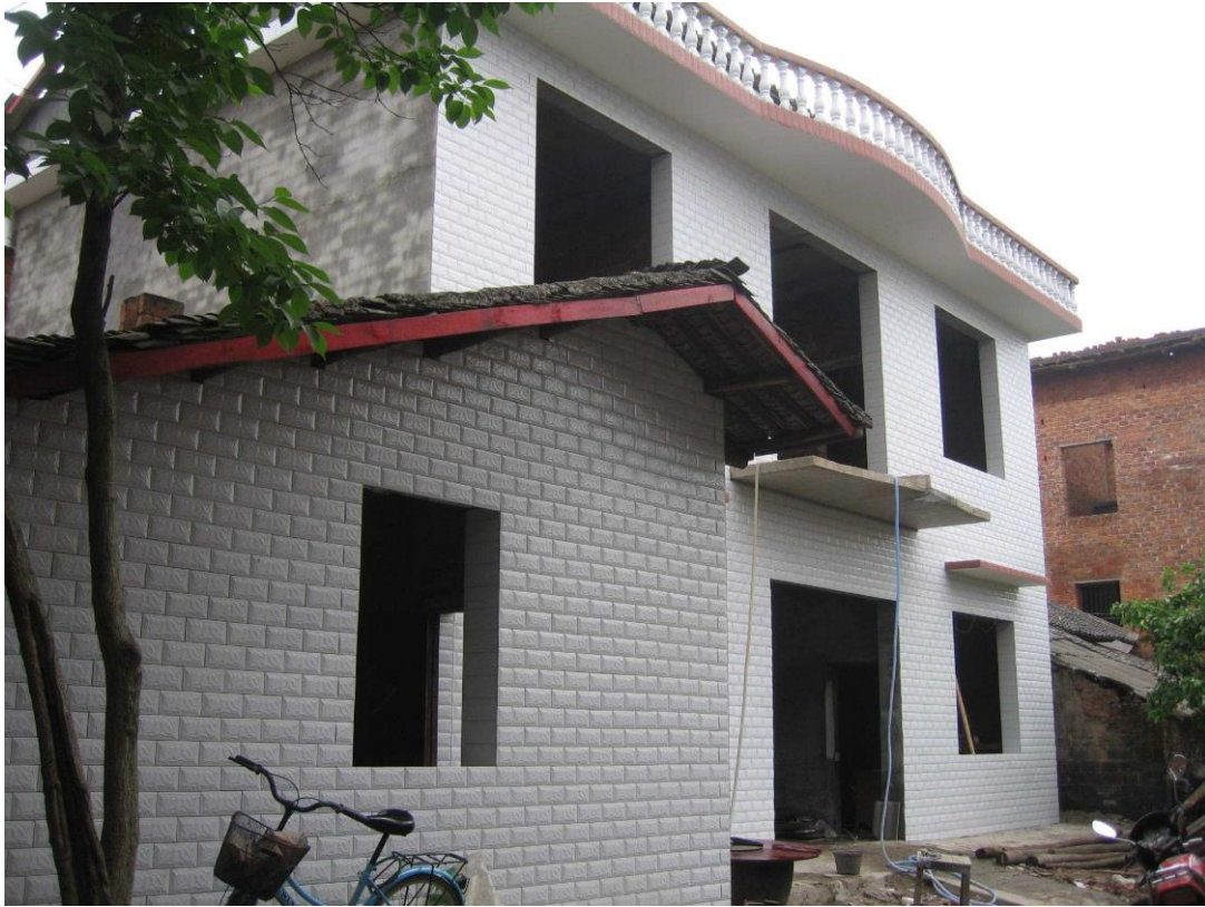
Figure 6.18 Son of the Yang couple's new house being constructed in 2009
