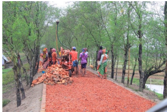
e. Rehabilitation of embankment (Polder 30)
