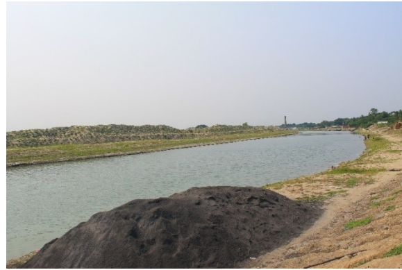
d. Excavated Kobedak River
