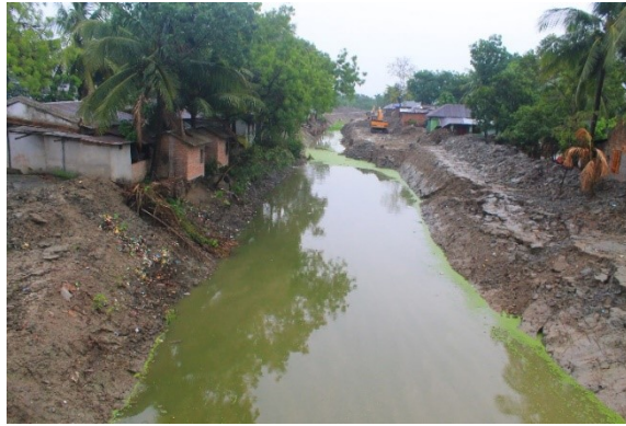
c. Excavation of drainage channel inside polder 29
