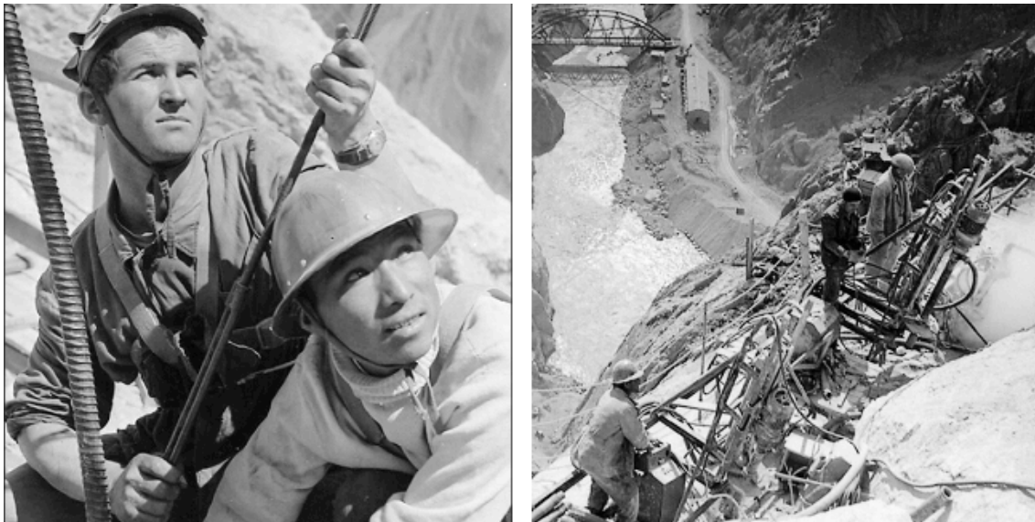
Figure 7.9 Photos of workers taken during the construction of the Toktogul dam. Young, healthy workers were often used as propaganda for socialism and these photos have been spread throughout the Soviet Union. Source: (Feaux de la Croix 2011).
