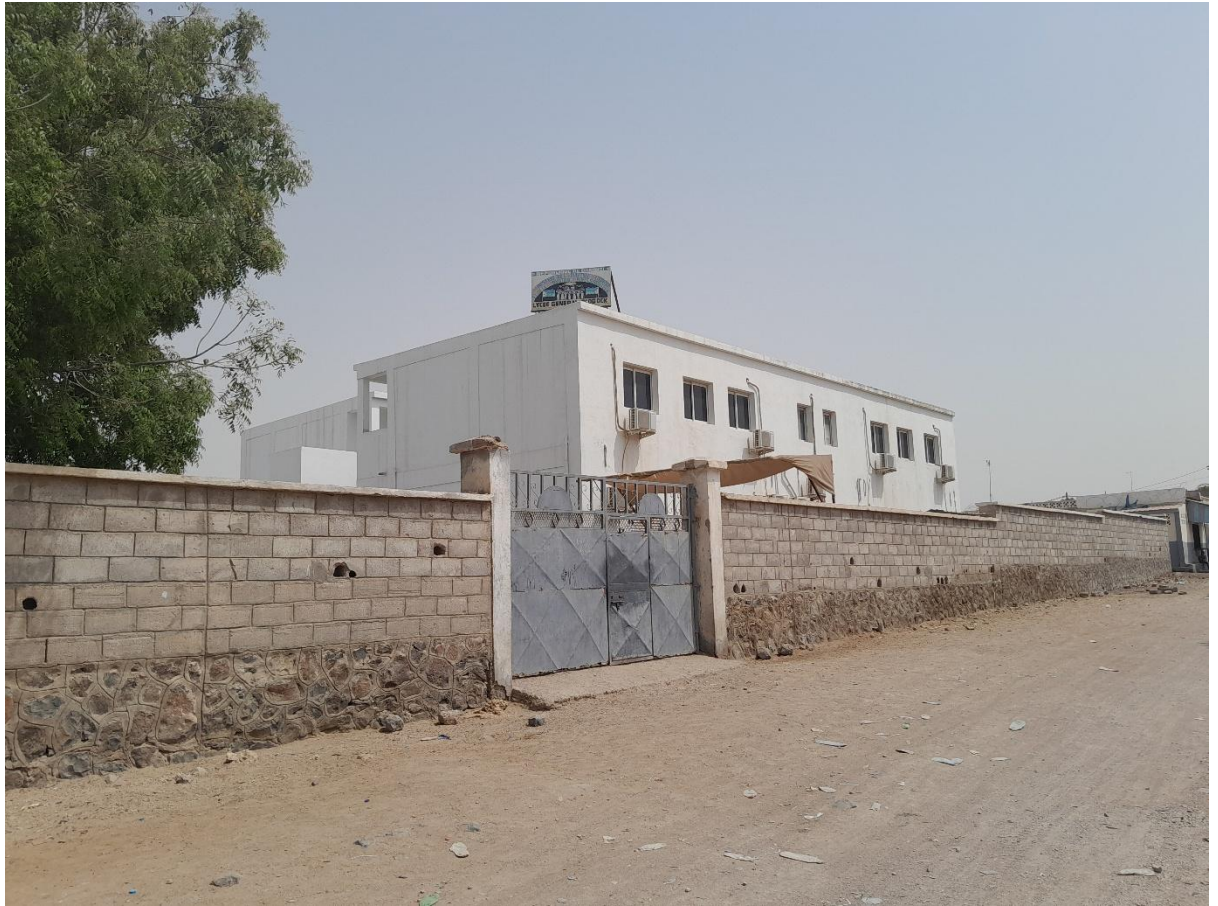
Figure 6: A wing of the local hospital built by smugglers.
