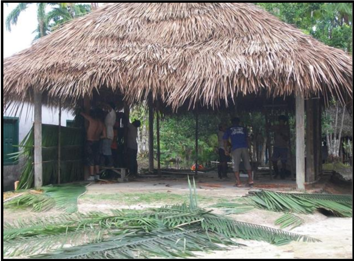
Figure 5: Carlos with the Tunu men thatching the walls of our house.
