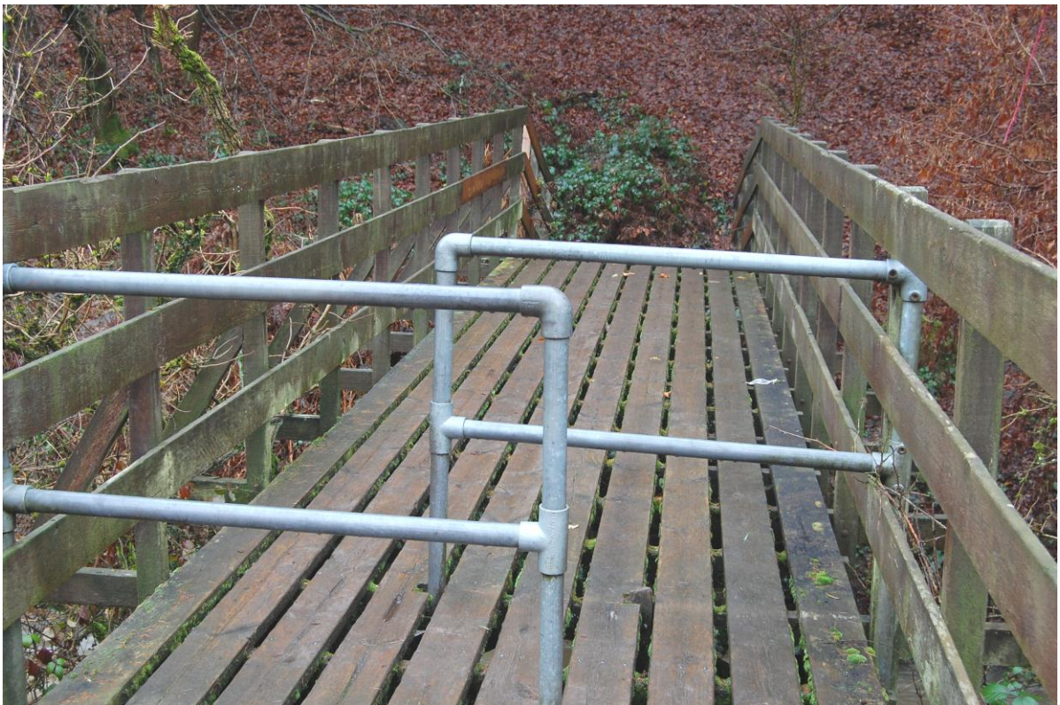
Figure 4.6: Footbridge to the Long Path, November 2008
