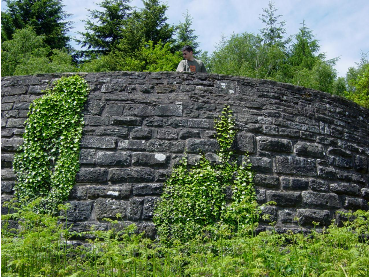
Figure 3.6: Retaining wall at Blaize Bailey Viewpoint, June 2006
