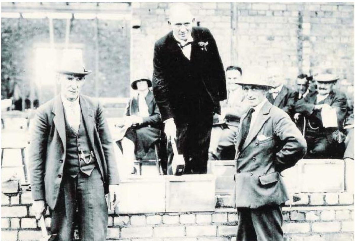
Figure 4.16: Laying one of the foundation stones of the Cinderford Miners' Welfare Hall, 1929 (Source: http://www.sungreen.co.uk/Cinderford/Cinderford-Miners-Welfare-Hall-1929.htm accessed 4 May 2010)
