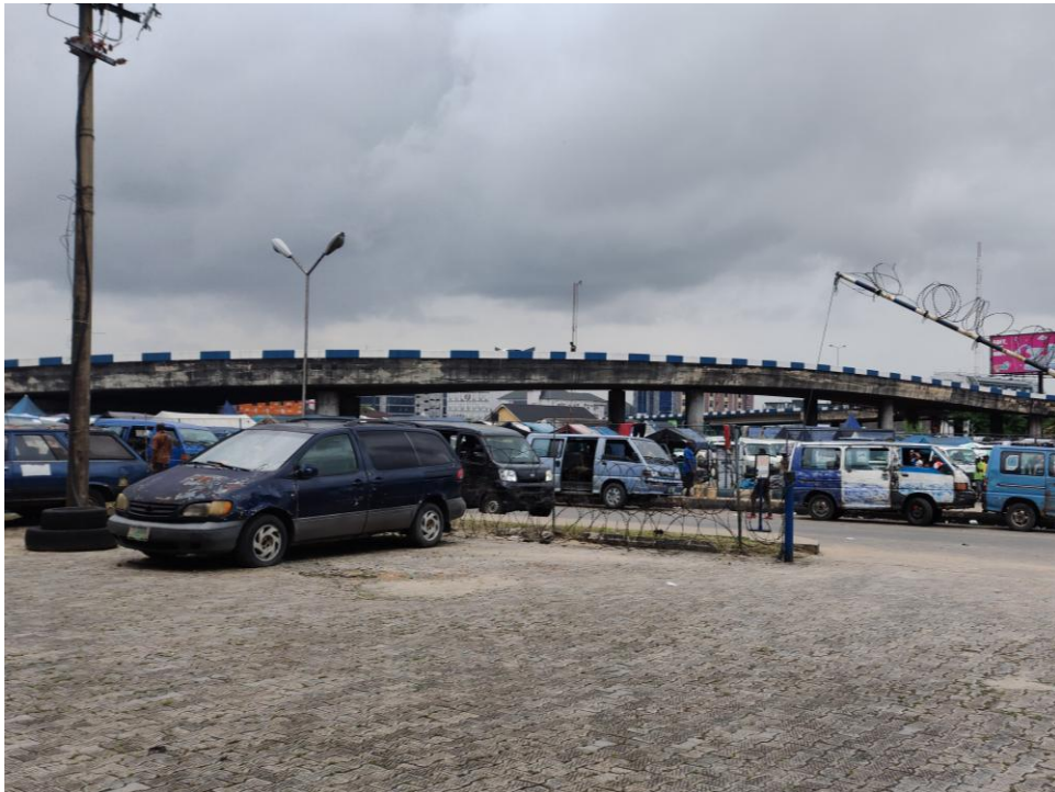
Plate 3: Mile 1 Diobu flyover
