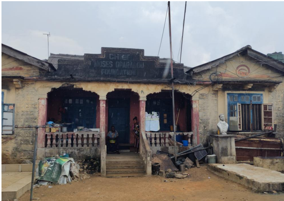
Plate 31: An Ikwerre bungalow in a compound in Ogbunabali (note the tombs)
