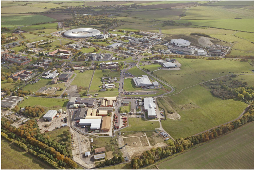
Figure 1.1: The Harwell Campus, including Rutherford Appleton Laboratory and the ISIS Facility
