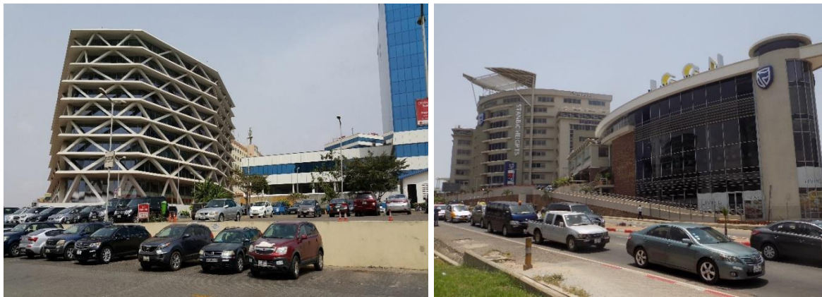
Figure 4. 6: One Airport Square (Left) and Icon House (Right)
