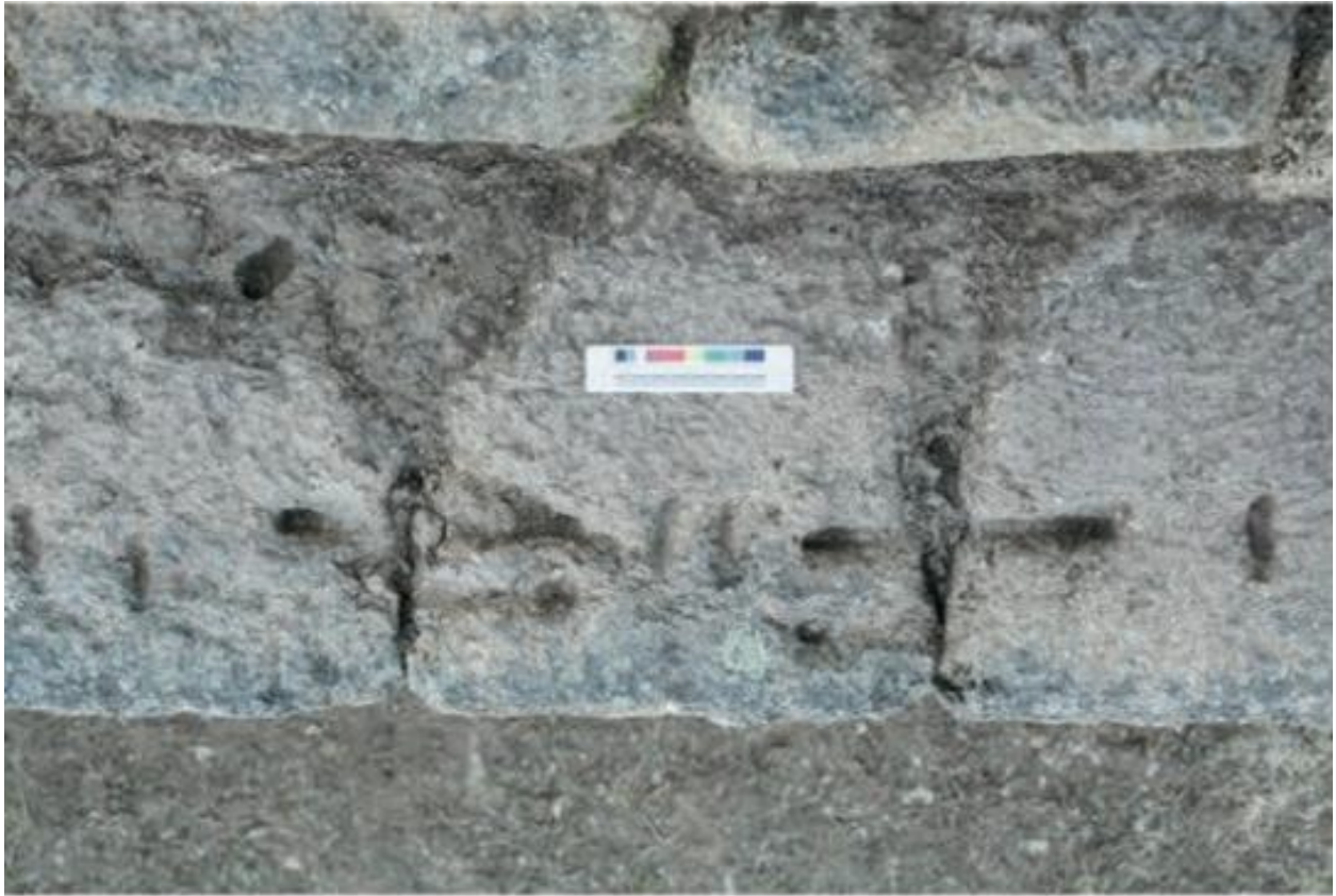
Figure 6.9: A section of ashlars with clamp holes from the crepis of Chetinyova (4) tumulus
