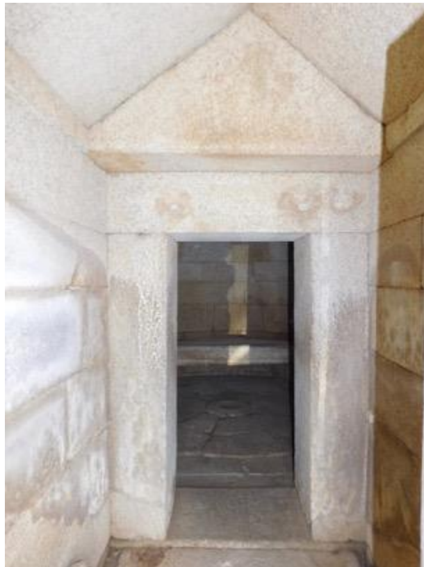
Figure 3.15: Holes for the metal rings used for holding the wings of the door of the burial chamber of the Golyama Arsenalka (17) tomb
