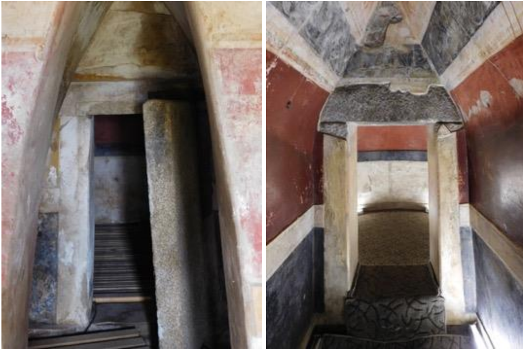
Figures 2.71 and 2.72: Stone lintels of the entrances to the burial chambers of Sarafova (L) and Kazanluk (R) tombs
