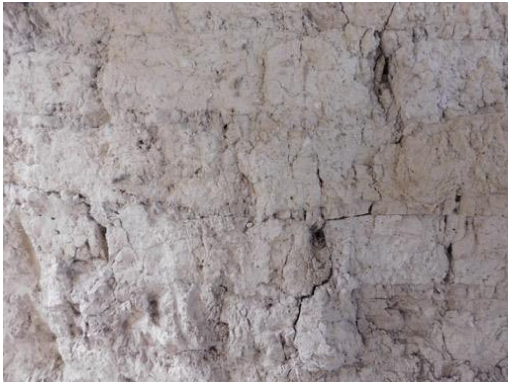
Figure 2.45: Section of the mudbrick construction of the dromos/façade of the Gagovo (68) tomb in 2019
