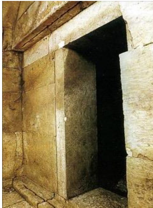
Figure 3.17: Detail from the interior of the tomb in tumulus 13 at Sboryanovo (71), showing the niches for the sliding door of the tomb
