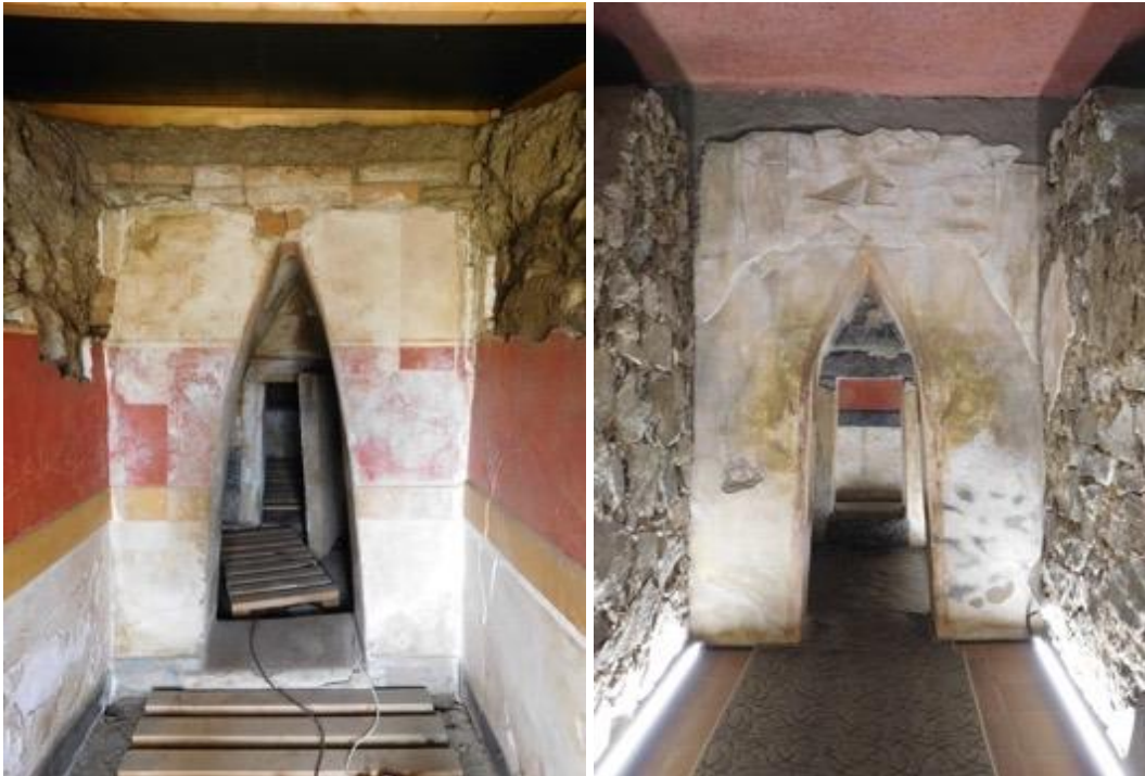
Figures 2.78 and 2.79: Main entrances to the (in order) Sarafova (26) and Kazanluk (22) tombs, made entirely of brick
