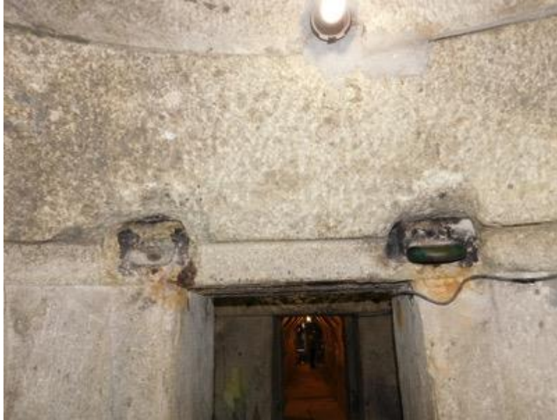
Figure 3.14: Metal rings used for holding the wings of the door of the burial chamber of the Mezek (41) tomb
