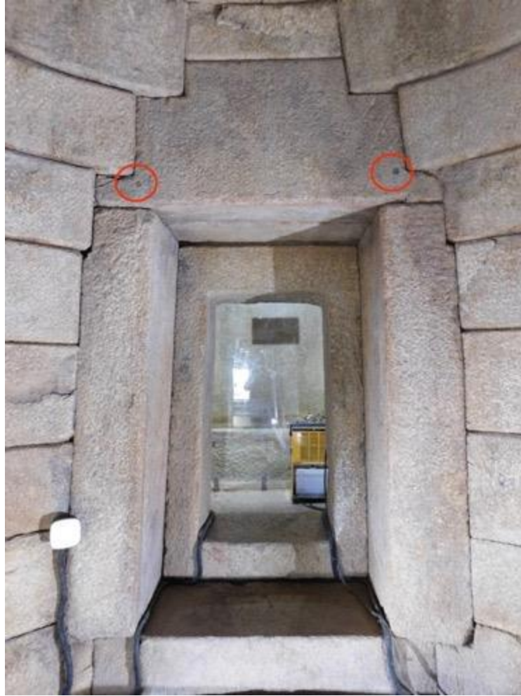
Figure 3.29: View of the entrance to the sarcophagus-like burial chamber of the Golyama Kosmatka (13) tomb, showcasing the holes used to attach the door
