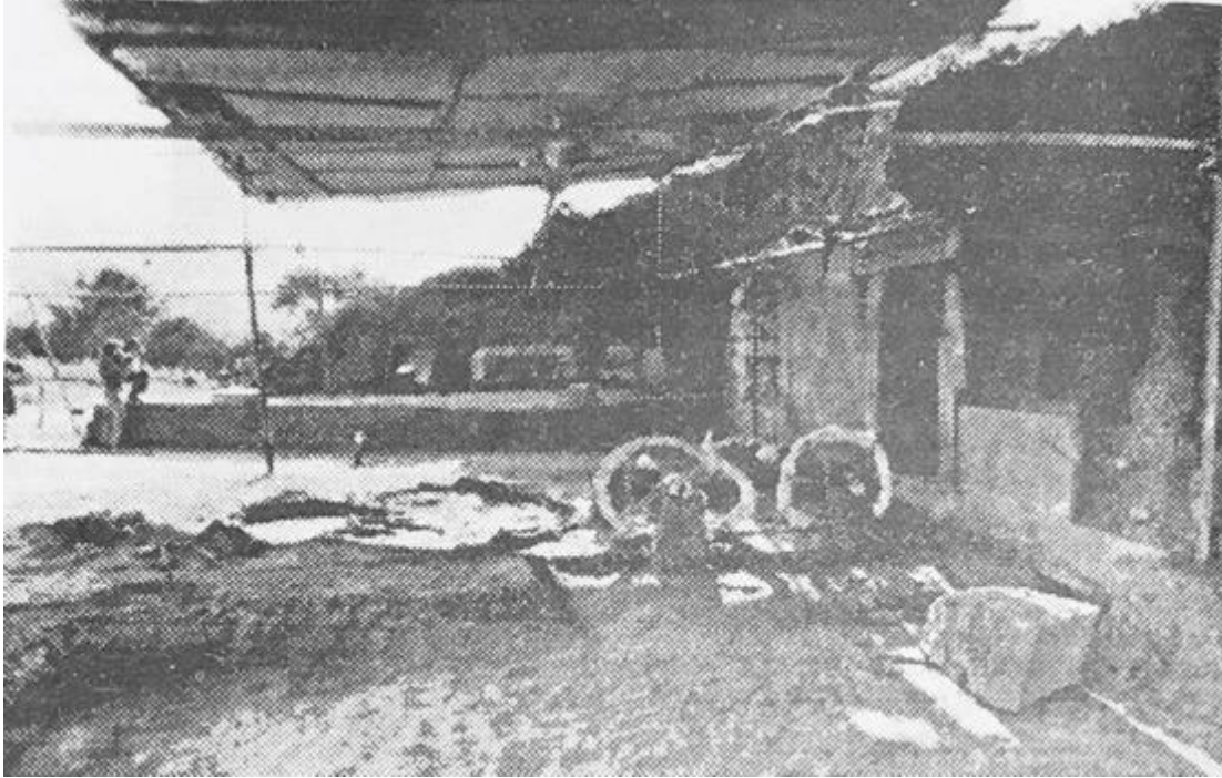
View of the façade and entrance of the Zhaba tomb with the chariot and horses in front of it at the time of discovery
