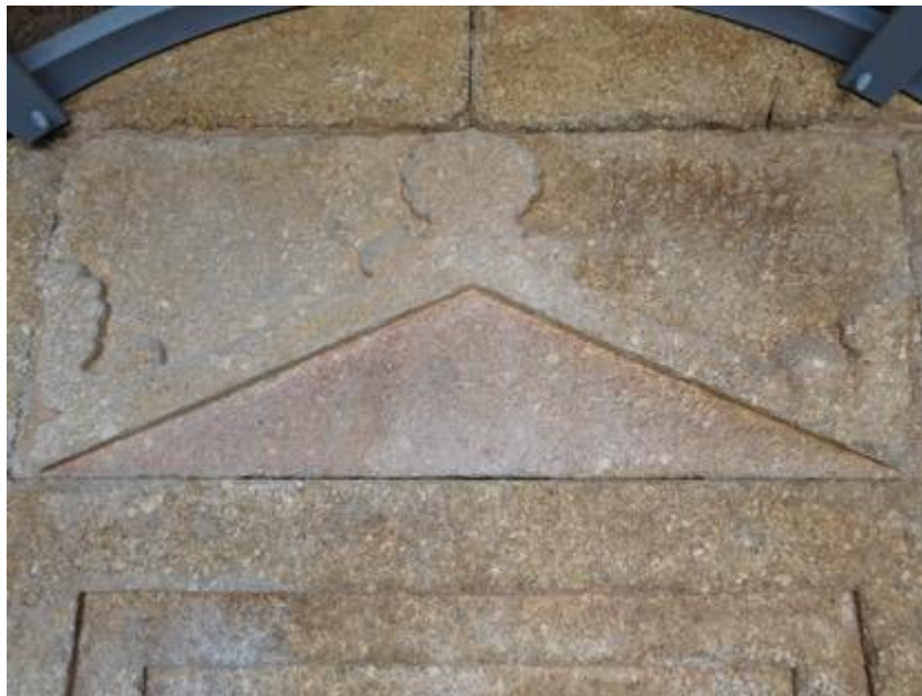
Detail of the entrance, showing the pediment and acroteria carved in relief
