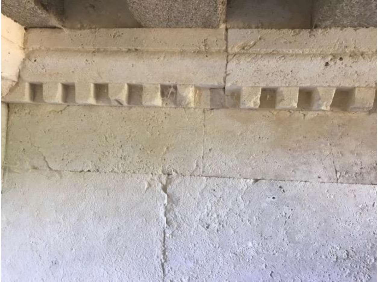
Detail from the interior, showcasing the beam-and-slab-type ceiling and decorative dentils below it
