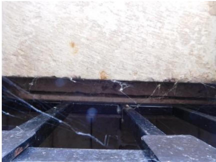
View of the entrance's lintel and the slot for the door on its interior side
