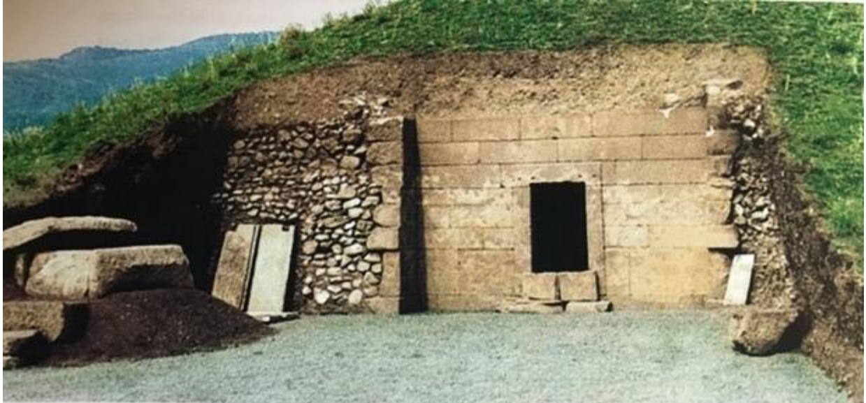
The façade of the Golyama Arsenalka tomb at the time of discovery with one cist grave visible to the left
