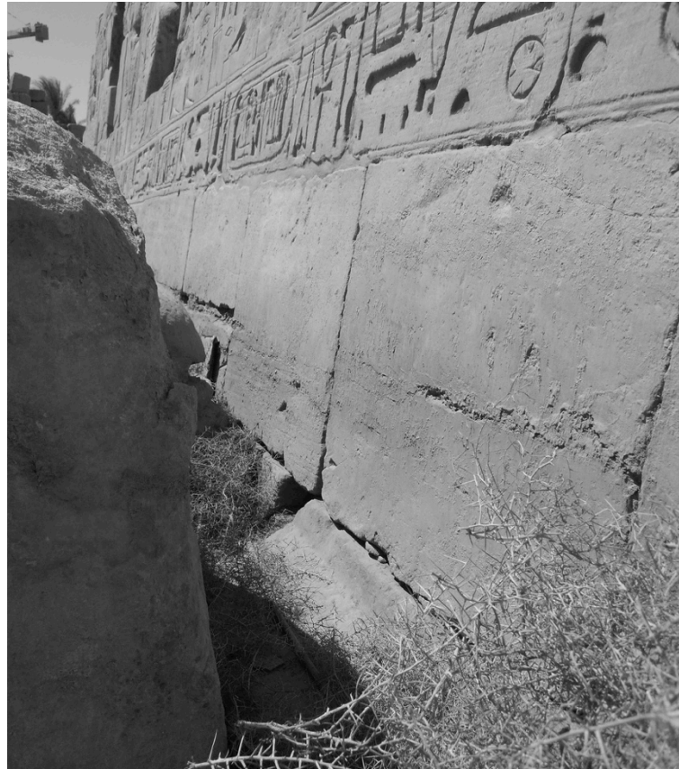
Fig. 3.8 Exposed foundation block of the interior west wall. © CNRS-CFFETK/C. Salvador.
