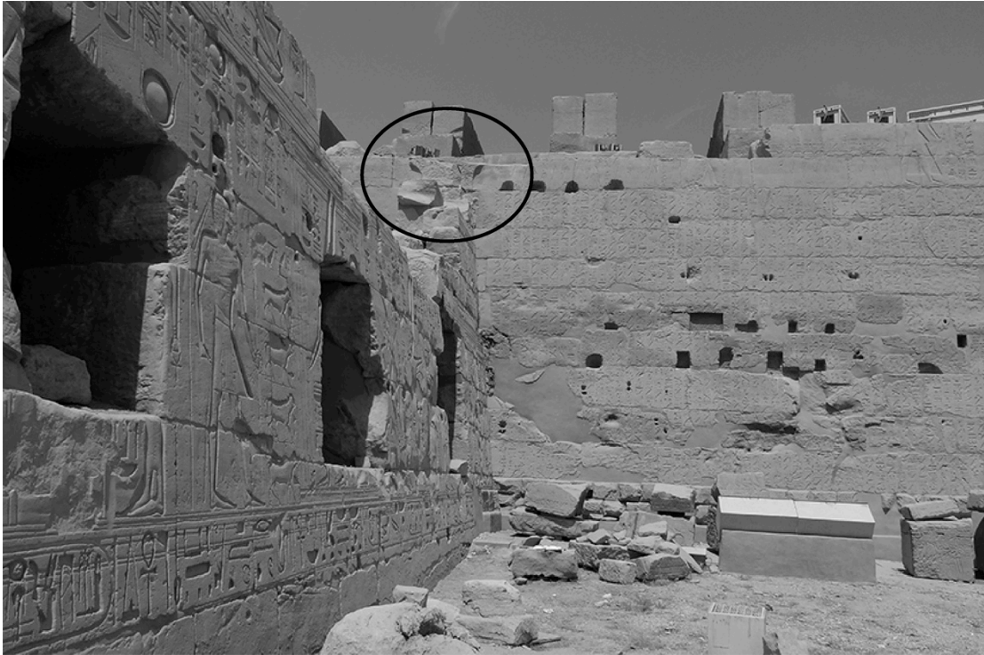
Fig. 2.5 The circle indicates the cavetto cornice of the north end of the west wall of CR7 embedded in the masonry of the south wall of the hypostyle hall, Amun temple, Karnak. © CNRS-CFEETK/C. Salvador.
