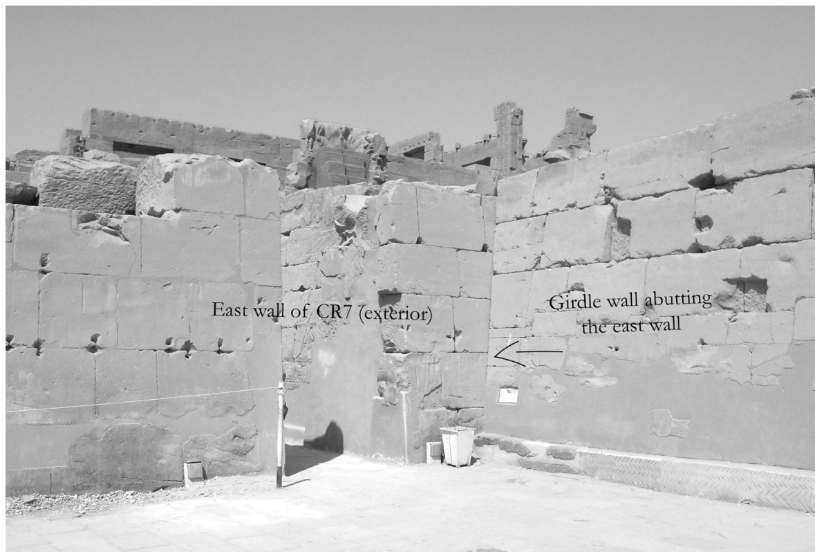
Fig. 2.6 The girdle wall of Tuthmose III abuts the north end of the east wall of CR7, also built under Tuthmose III but slightly earlier. © CNRS-CFEETK/C. Salvador.
