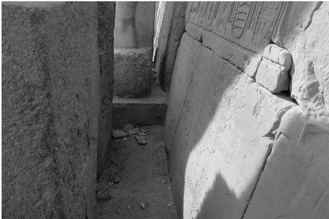
Fig. 5.2 View from the west of block A1 on the west massif of the seventh pylon (to the right) hidden behind the rear of two seated statues (PM II 2 : 168 (E–F)).
