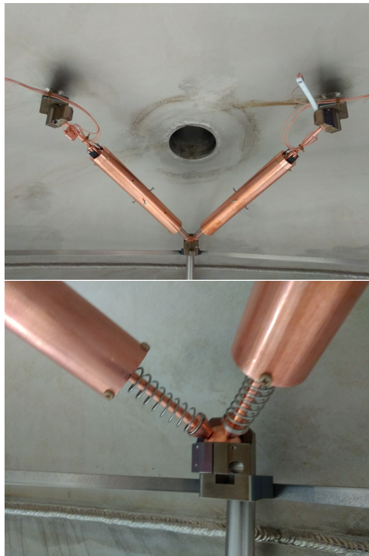
Figure 5.6: (Top) An example of a corner triangular arrangement. This image is taken with the vertical calibration rods installed (very bottom of the image) which mimic where the top array would sit during initial installation. (Bottom) Springs seen at the ball joint were added to ensure that the bottom hexagon maintains a good attachment to the top array.
