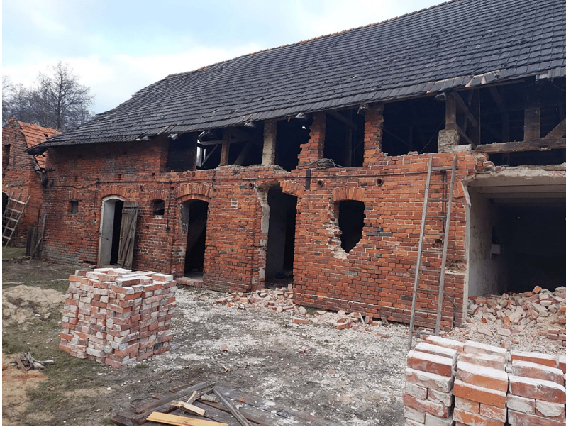
Figure 1. ‘Restruction’ of an agricultural building for the extraction of circular building materials. © DolveVita, BauXpert Gebhard GmbH & Co. KG, with friendly permission.
