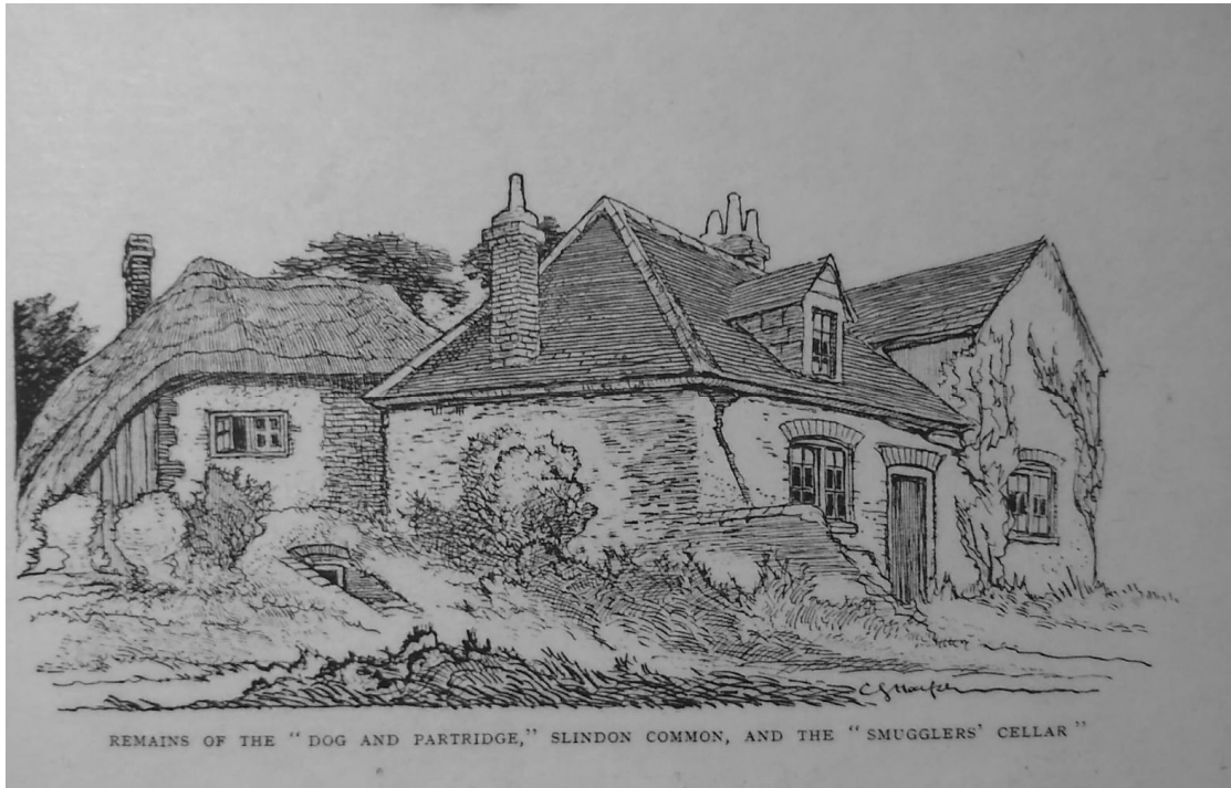
Figure 4.4 Sketch of a pub where a hull (bottom left) is identified as a Smugglers Cellar (Jamaica Inn Museum 2021).
