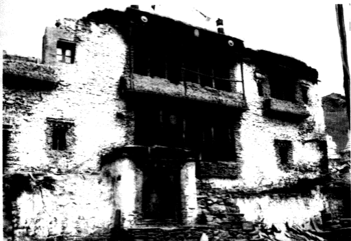
2. Korzok Gompa, while renovations were in progress, in 1993.
